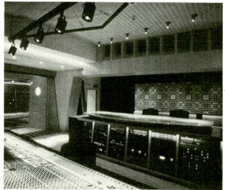
The Russ Berger-designed control room at Whitney Houston's home studio, featuring the first-ever-built SSL 9000 console, Studer 48-track digital and 24-track analog recorders, and RPG diffusor blocks.
