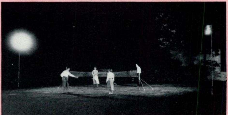
In badminton, two of the three-lamp, 12-foot poles are used, located on the net line 15 to 20 feet from the net. Equipped with 300-watt floods, these provide ample light for following birds.
