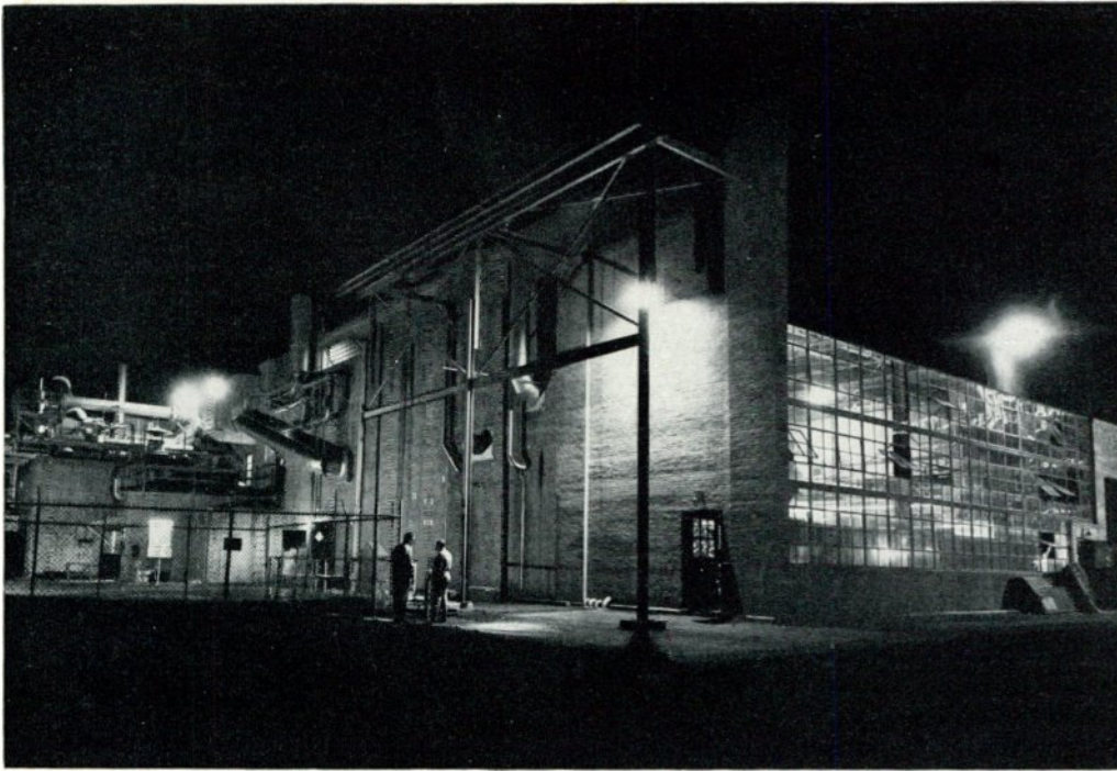
The laboratory is built on the banks of the Saugus River, a tidal inlet. At the rate of 80,000 gallons per minute, water is channeled into the building for cooling purposes. Channel is at left behind fence.
