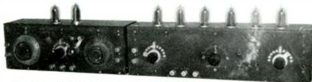
ARMSTRONG'S SUPERHETERODYNE TUNER AND I-F AMPLIFIER 1918
