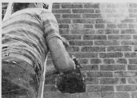
Fig. 8. The final trim is done by hand with a cold chisel and small sledge. The sheet metal duct should just slide through the hole without bends or a force fit. Chip away small bits of brick until the duct can slide in and out easily.
