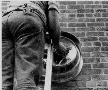
Fig. 11. Install the motor, making certain the BX cable armor runs all the way to the motor connection box to provide a solid electrical ground. If you're using Romex wire make certain you use the type with the ground wire, and double-check that the ground is secure at the motor.
