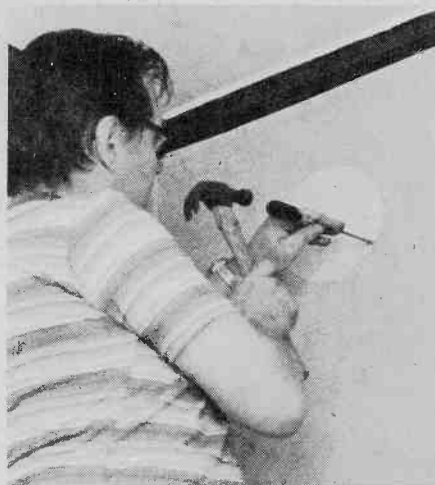
Fig. 2. If the wall is sheetrock (drywall) score the outline with a knife, a narrow chisel, or an old screwdriver, then cut all the way through and punch out the circle.
