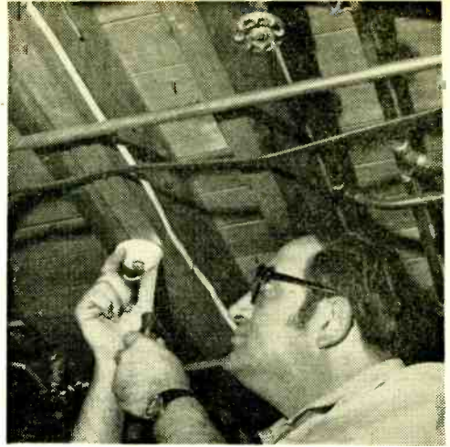
Standard open circuit heat/fire detectors can be installed in all living areas, above the furnace and in cellar and attic.
