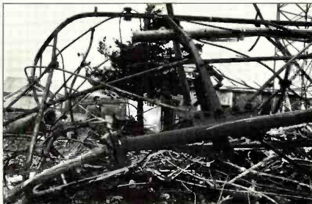
**Tower trouble.** The 2,000-foot broadcast tower of Allbritton Communications' KTUL-TV Tulsa, Okla., collapsed on Saturday, Dec. 26, during an ice storm. The station remained black for nearly 24 hours after the incident. Said Jerry Fritz, head of engineering for Allbritton, "It's clearly a tragedy on our part but fortunately no one was hurt."
