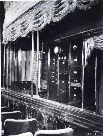
A VIEW OF THE CONTROL ROOM OF THE COLUMBIA RADIO PLAYHOUSE, SHOWING THE MIXER CONSOLE AND EQUIPMENT RACKS. RCA VICTOR STUDIO EQUIPMENT USED THROUGHOUT
