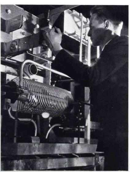
JOE CHAMBERS CLOSING A FILAMENT SWITCH IN ONE OF THE POWER AMPLIFIERS.
