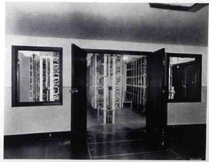
VIEW LOOKING INTO THE MAIN DISTRIBUTING FRAME ROOM SHOWING THE THREE FRAMES WHERE ARE TERMINATED 1250 MILES OF WIRE
