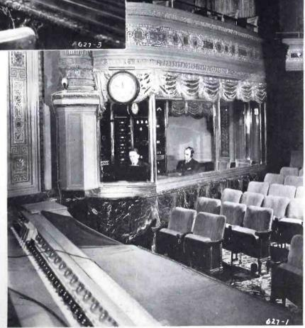
CONTROL ROOM OF COLUMBIA RADIO PLAYHOUSE, BUILT INTO THE ORCHESTRA BOX SECTION AND BEHIND DOUBLE-GLASS PANELS. THE EQUIPMENT RACKS ARE SEEN IN THE BACKGROUND, THE MIXER CONSOLE IN THE FOREGROUND. RCA VICTOR STUDIO EQUIPMENT INSTALLED THROUGHOUT
