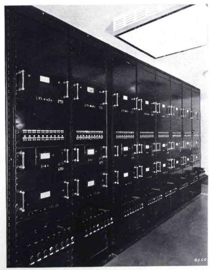
VIEW SHOWING SOME OF THE RACKS AND AMPLIFIERS LOCATED IN THE EQUIPMENT ROOM. AMPLIFIERS SHOWN ARE STUDIO, TALK-BACK, ISOLATION AMPLIFIERS SUPPLIED TO NBC BY RCA VICTOR CO., INC.
