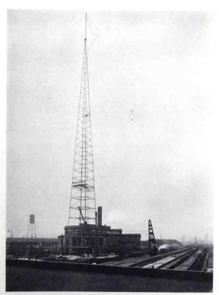
ANTENNA OF STATION WJY, AT THE LACKAWANNA RAILROAD TERMINAL IN HOBOKEN, N. J. THE RADIO TOWER, WHICH IS STILL STANDING, WAS ORIGINALLY BUILT AS PART OF THE LACKAWANNA'S RADIO TRAIN DISPATCHING SYSTEM, AND ENABLED THE ROAD TO KEEP TRAINS RUNNING DURING BLIZZARDS THAT CRIPPLED WIRE COMMUNICATIONS AND COMPLETELY PARALYZED OTHER ROADS IN THE DISTRICT. SIMILAR STATIONS WERE LOCATED ALONG THE LINE AT BINGHAMTON, SCRANTON AND BUFFALO
