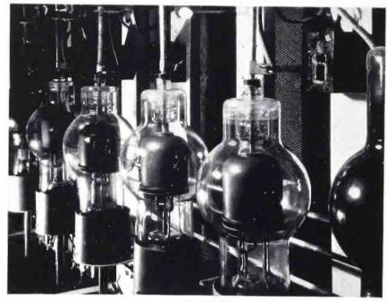
THE RCA-870 TUBES IN THE MAIN RECTIFIER. THESE AIR-COOLED TUBES HAVE AN ANODE CURRENT RATING OF 450 AMPERES AND HAVE AN ACTUAL EMISSION OF ABOUT 1,500 AMPERES EACH. YET THE POWER REQUIRED BY EACH CATHODE IS ONLY 325 WATTS
