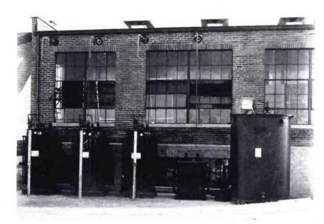
THIS VIEW SHOWS THE MAIN PLATE TRANSFORMERS, FILTER REACTOR, AND MODULATION TRANSFORMER
