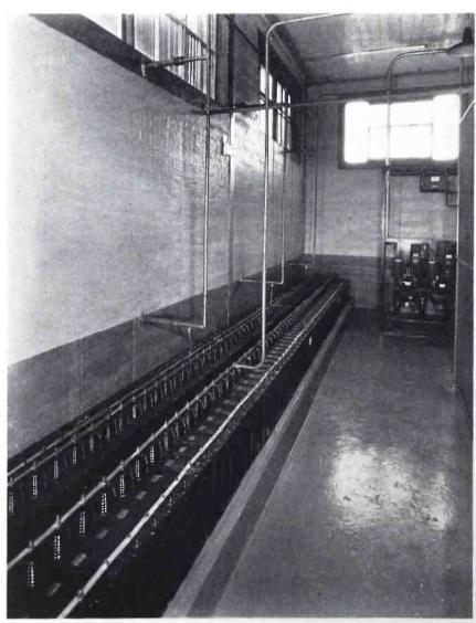
THE FILTER CONDENSER OF THE MAIN RECTIFIER HAS A CAPACITY OF 220 MFD. WHEN THIS CONDENSER IS CHARGED TO 12,000 VOLTS AND THEN SHORT-CIRCUITED, THINGS HAPPEN.
