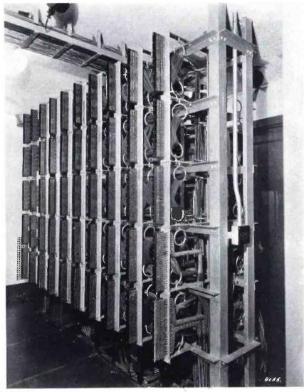
THIS VIEW SHOWS A CLOSE-UP OF ONE OF THE THREE MAIN DISTRIBUTING FRAMES WITH THE TERMINATION BLOCKS AND METHOD OF HANDLING THE WIRES AND CABLES TO THE BLOCKS
