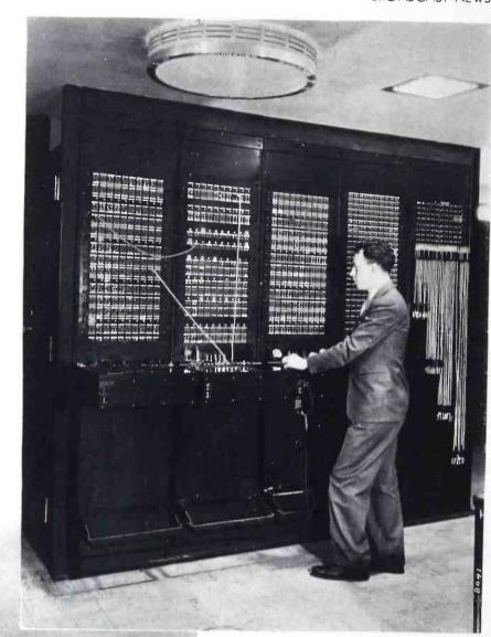
(ABOVE) LINE TERMINATING RACKS LOCATED IN THE MASTER CONTROL ROOM
