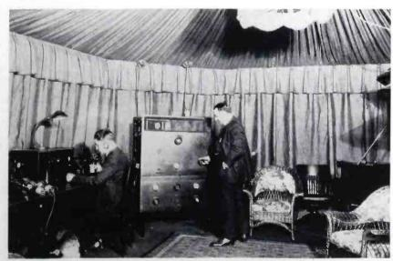
STUDIO AT WDY, ROSELLE PARK, N. J. 31/2 KW. BASE STATION SET IN CENTER. NOTE WICKER FURNITURE AND ELECTRIC HEATER AT EXTREME LOWER LEFT. AN UPRIGHT TELEPHONE TRANSMITTER, SUPPLIED WITH THE SET, WAS USED AS A MICROPHONE
