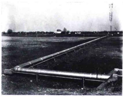
THE LARGEST AND LONGEST CONCENTRIC TRANSMISSION LINE IN THE WORLD. THIS 820-FOOT CONCENTRIC LINE, WITH AN OUTSIDE DIAMETER OF 10 INCHES, IS KEPT NEAR THE GROUND, AND GROUNDED EVERY 20 FEET, TO PREVENT HARMONIC RADIATION. THE CONSTRUCTION IS SUCH THAT ANY OF THE MYCALEX INSULATORS WITHIN THE LINE OR ANY SECTION OF THE LINE MAY BE REPLACED IN A FEW MINUTES TIME.
