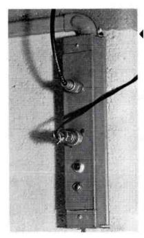
FIG. 13. Classroom TV control stations showing RF and receiver muting cables, talk-back pushbuttons, and technician phone jacks. (Left) Surface mounted. (Below) Flush mounted,
