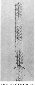
FIG. 9. The RCA BFA-12A center-fed antenna is corner mounted on one of 445-toot AM towers. At the bottom of the FM antenna the transmission line can be seen as it swings into the tower. From this point the line is supported at the cross bracing that carries the ladder, making the line readily accessible for inspection.
