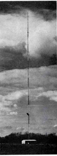
FIG. 33. WAVE-TV transmitter site 500 feet above Louisville. The tower and TF-6AL Antenna overall height are 600 feet. The location, Bald Knob, Indiana, is the highest site in the Louisville area for television towers.
