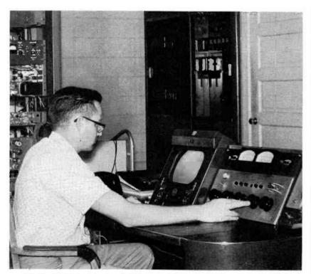
FIG. 12. WTVM transmitter plant. In foreground is the TTC-5 Control Console. At far background are the rectifier and control cabinets for the TT-25CH aural power amplifier.
