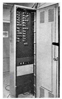
FIG. 14. College of Education talk-back control rack. Contains audio line amplifier, RF amplifier, relays and associated circuitry.
