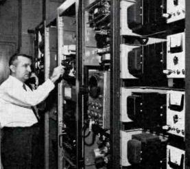
FIG. 37. An RCA STL microwave unit is adjusted by Robert Roth, maintenance and equipment supervisor in Louisville studio building. Rotatable antenna on tower is also controlled here.
