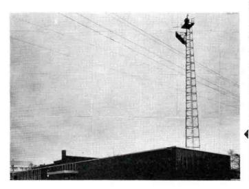
FIG. 36. Self-supporting 135-ft. microwave tower. Note two receiving dishes on platform—one fixed, and one rotatable. The reflector handles a 7000 mc STL microwave and also a 2000 mc STL, both with roof-mounted
