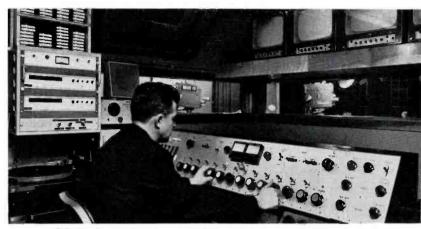
FIG. 21. Roy Parris at audio console in studio control room. It's duplicate of control in equipment room. Both were built by WAVE-TV. All amplifiers are housed in cubicle under console. At left is RT-7A Cartridge Tape unit.
