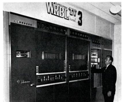
FIG. 8. WRBL-TV employs 25-kw Type TT-25CL TV transmitter.
