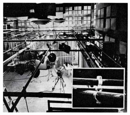
were bolted into the ceiling. The ceiling height is 21 feet. The pipe grid is 13 feet above the floor. Rectangular electrical duct was fastened to the steel rods just above the pipe grid. There are 22 electrical circuits in these ducts for lighting and all circuits are controlled by low-voltage relays. A special switching circuit makes it possible to control as many of the individual circuits from a single switch as is desired. Figure 5 shows the pipe grid with all lights.
