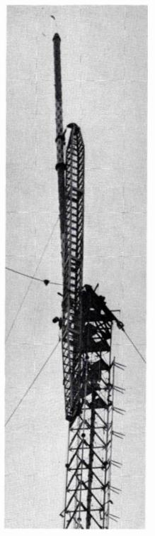
FIG. 3. The RCA TFU-46K as it went into place atop the tower. Capable of a power input of 110 kilowatts, the antenna delivers an ERP of 480 kw with a 12.5-kw transmitter. Driven with 110 kw of peak-visual power, the antenna would radiate 5 megawatts. ERP.
