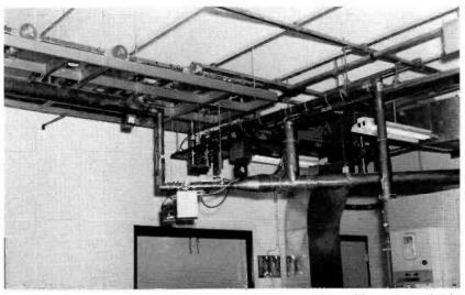
FIG. 5. This view of the RCA transmitter shows the side band filter, ceiling mounted visual low-pass filter, co-ax patch panel and gassing system for exterior coax run. All this was installed at the new WOW-TV transmitter building.
