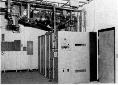
FIG. 4. This view shows the rear of the transmitter with the transmitter enclosure, hybrid couplers, visual low pass filter, tower light indicator panel and other vital parts.
