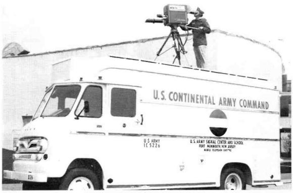
FIG. 2. Mobile van with cameras, TV tape and microwave link makes remote pickups for instruction and troop entertainment.
