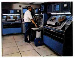
Camera control area is spacious and uncluttered. Engineer Don Bednarek rides video on one of the six TK-44B cameras operated from this position. Console also Includes controls for 1—TK-28 Film System; 1—TK-27 Film System, as well as Pulse assignment and Genlock. Intercom system is a BCS-5000.
