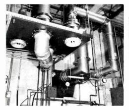
Manual coaxial patch panel for 9A-inch transmission line to antenna.
