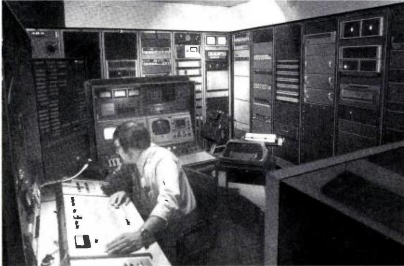
Master Control is unusual in that video and audio equipment racks form two of its walls. The racks back on the engineering shop space, for service accessibility.
