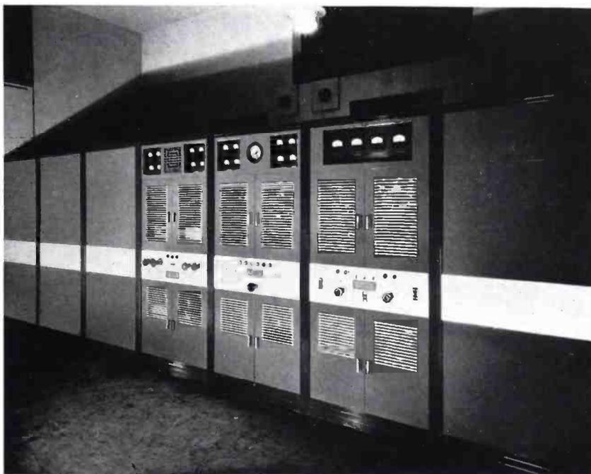
The New RCA 5-C, 5 KW transmitter installed at WFBC.
