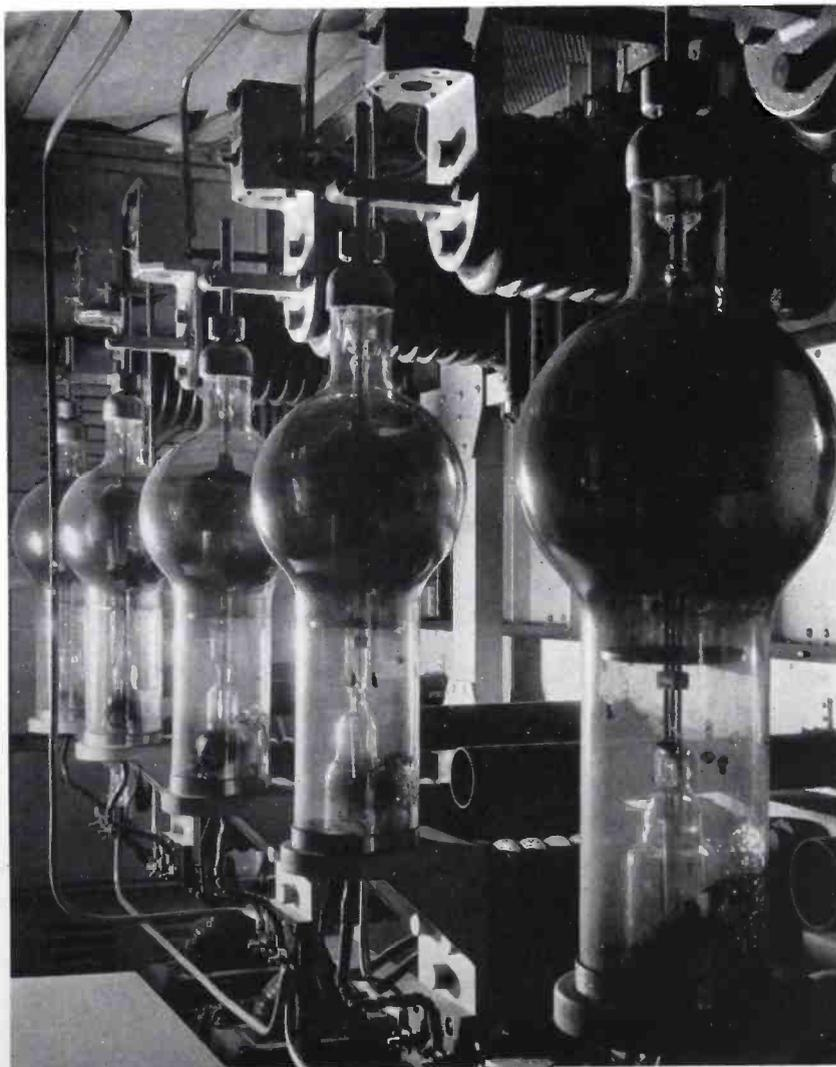
Lineup of rectifier tubes in the 50-C.
