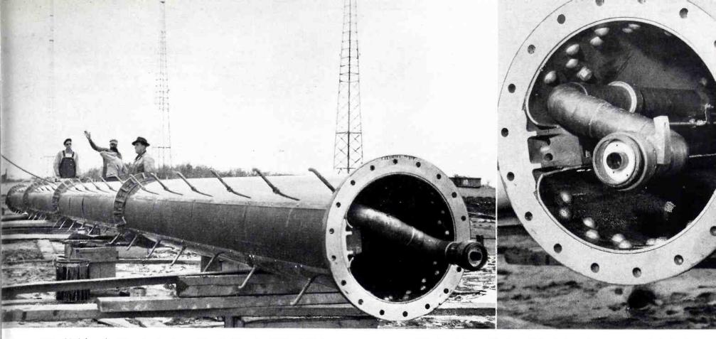
FIG. 11 (above). Here is the top unit—oll four standard aluminum sections bolted together and complete with transmission line installed and tested.
