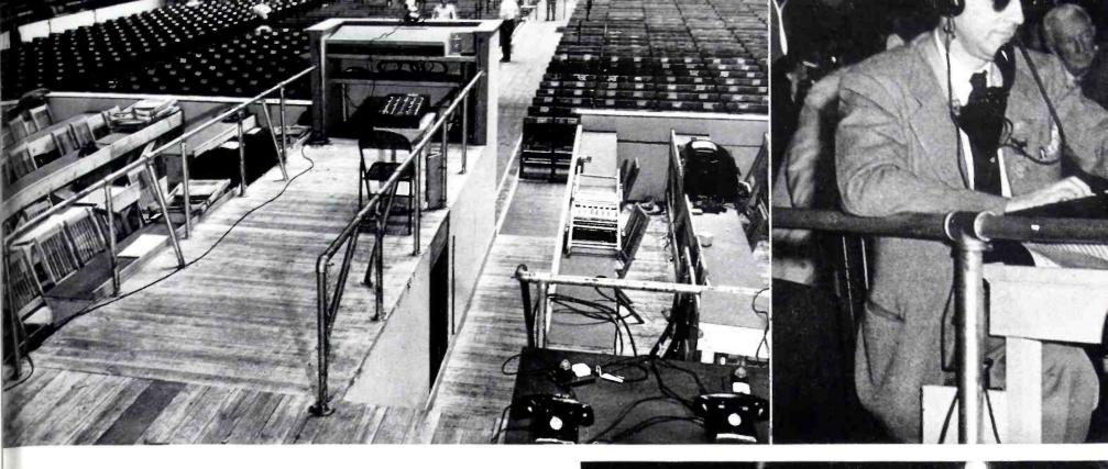
MICROPHONE SWITCHING is an extremely important operation in the conduct of a big convention. The small black box on the table just back of the rostrum (above) contained the switches controlling the floor microphones. A technician sitting at this position (right, above) could connect any floor microphone into the public address and radio systems at the direction of the convention chairman, and disconnect it just as quickly. This control of the situation was a powerful tool for the chairman.
