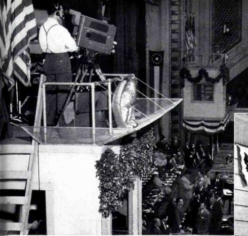
NO. 5 CAMERA POSITION (at right) was on a mobile TV unit just to the right of the main entrance. This was used just before meetings to show delegates arriving. Truck is an RCA Type TJ-50A Mobile Unit; Cameras are RCA TK-30A's. Equipment was furnished by ABC and operated, for the pool, by ABC technicians.
