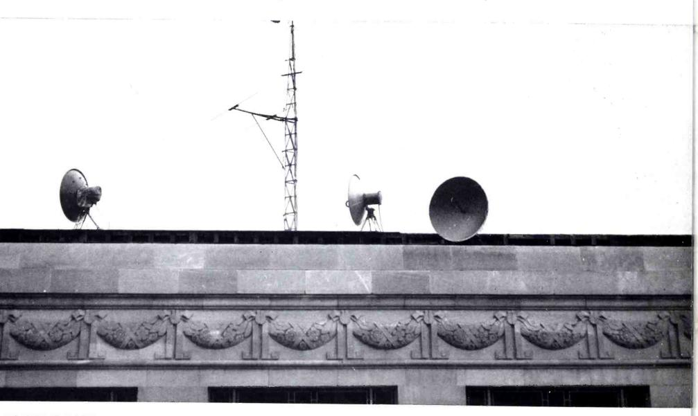
MICROWAVE RELAYS, most of them using standard RCA equipment units, were employed between the various pickup points in Philadelphia. Parabolas on the roof of Convention Hall are shown here. The two on the left are, NBC and ABC receiver units on line from the hotel. Parabola on right is NBC transmitter unit directed to relay system terminal at Wyndmoor. Structure on tower is old low-frequency antenna.
