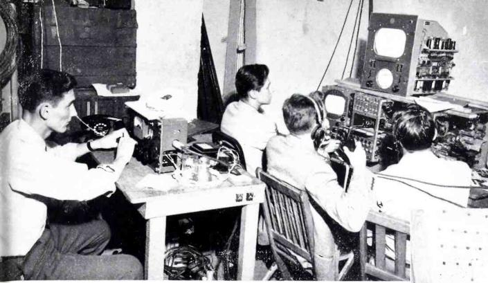
NBC's HOTEL CONTROL ROOM is shown at the left. Video units (at right of picture) include two RCA TK-30A Camera Cantrol Units, with a TS-30A Switcher between, and a TM-5A Master Monitor on top. Audio position, at left, features an OP7.
