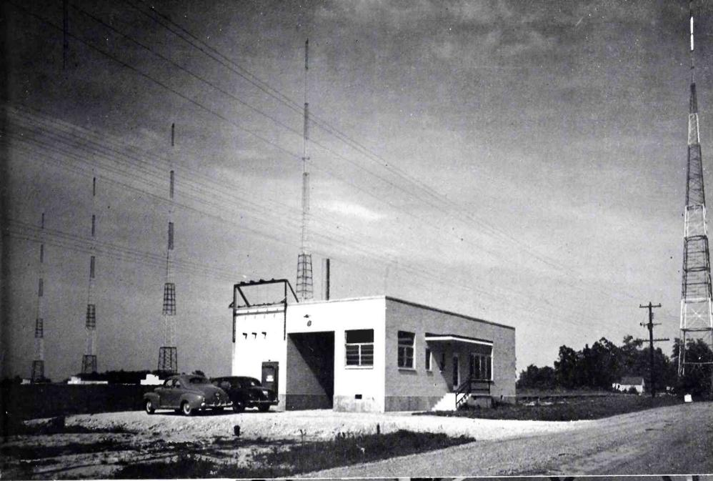
FIG. 2 (above). Here is the WKJG-FM and AM transmitter building and towers. Visible in the background is the WKJG AM antenna array—at the far right is the eight-section Pylon.
