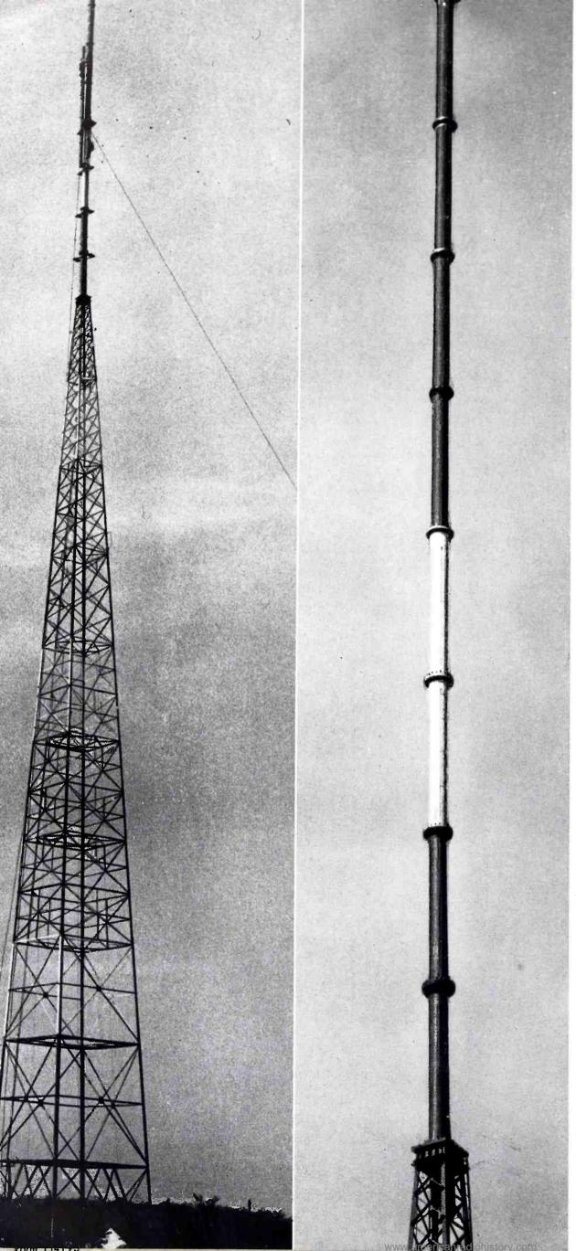
wind which delayed erection of the top four sections ceased about five o'clock one morning and the top four sections were hoisted and fastened into place, including transmission line connections, in less than two hours.
