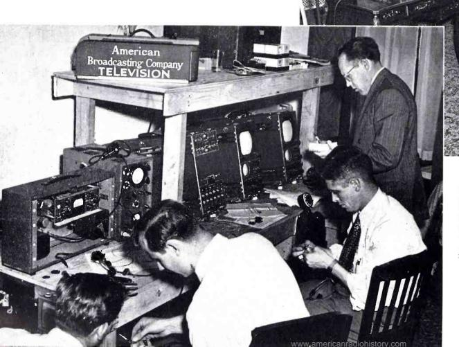
ABC's HOTEL CONTROL ROOM, shown at left during installation, was furnished with standard RCA TV equipment. Units shown are, from left to right, TTR-1A Microwave Transmitter (control only), WO-79A Oscilloscope, TS-30A Switcher, and two TK-30A Camera Controls. On the shelf above, only partly visible in this view, is a modified RCA receiver used as a master monitor on the outgoing line.
