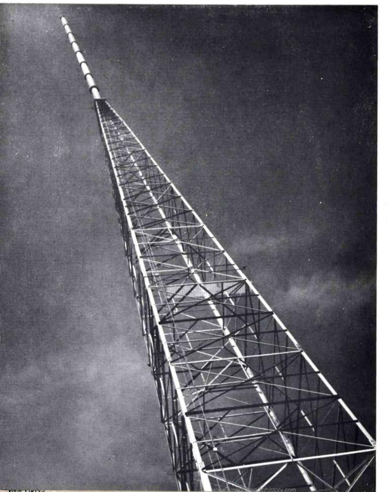
FIG. 1 (at le<sup>4</sup>t). Rising to a total height of 369 feet, the new "Super-Power" eight-section Pylon antenna provides an effective radiated power of 30 kilowatts.
