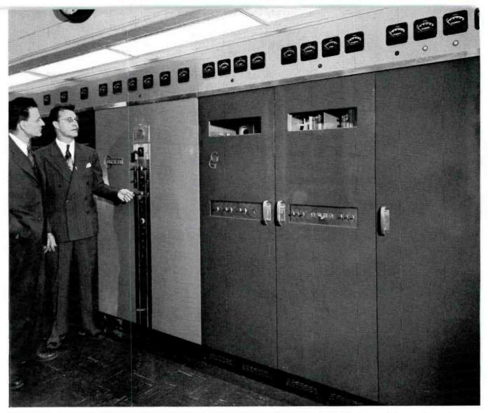
FIG. 2 (above). WBRC-FM's 50 KW transmitter, RCA type BTF-50A, presents a streamlined appearance, with all essential controls front-panel mounted and easy to reach. In this view G. P. Hamann, author, is at the controls while C. J. Starner, RCA engineer, looks on.
