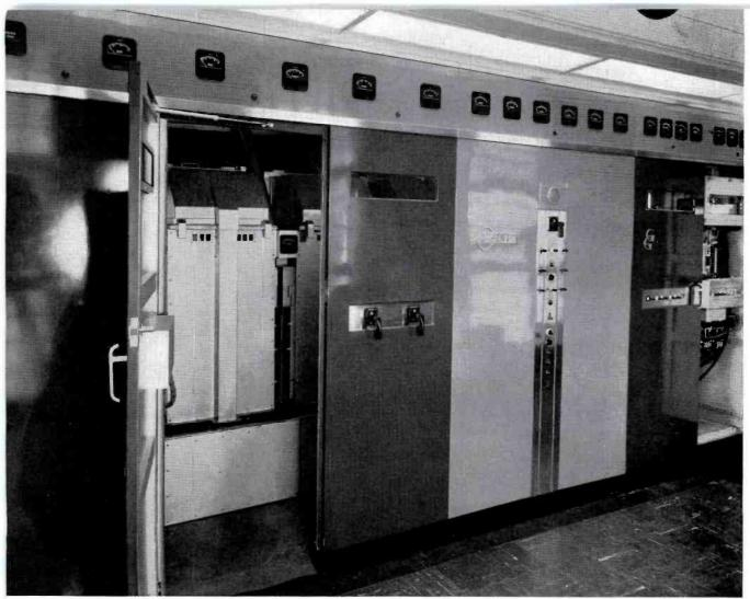
FIG. 3 (above). Front view of the WBRC-FM transmitter with doors opened to illustrate extreme accessibility. Note how 50 KW tanks at left are mounted so as to provide walk-around space.
