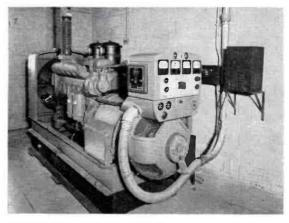
FIG. 8. To insure uninterrupted broadcast service, WMPS installed this 60 KW Diesel auxiliary generator for use in case power fails.
