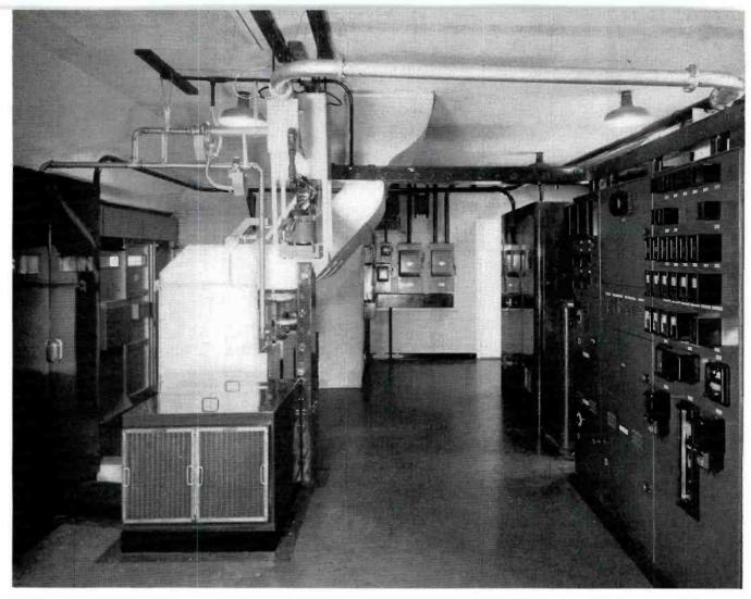
FIG. 5 (above). This view shows the entire BTF-50A. 50 KW FM enclosure. Low power r-f and exciter are at left. 50 KW grounded-grid amplifier at left center, and H-V rectifier and power and control units at the extreme right. Plenty of walk-around space is provided for every unit of the transmitter.
