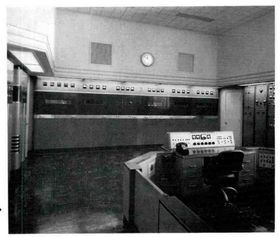
FIG. 2. The station is as neat looking inside as outside. Shown at right is the transmitter room which contains a 10 KW RCA Type BTA-10F Transmitter, a 1 KW BTA-11 Standby Transmitter, the speech input equipment, and the operator's control console.
