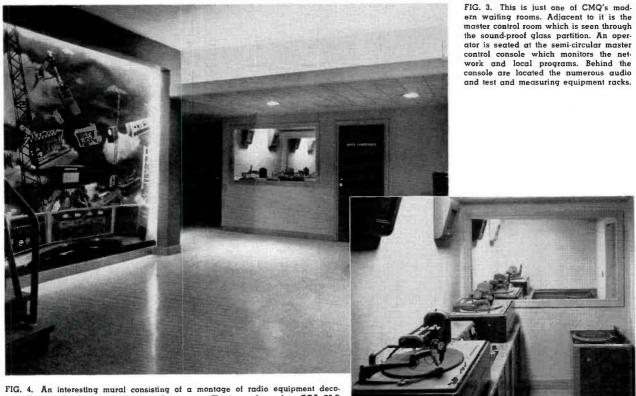
FIG. 4. An interesting mural consisting of a montage of radio equipment decorates the corridor leading to the recording rooms. The inset shows four RCA 73-B Professional Recorders and 70-D Transcription Turntables which are used by CMQ in its deluxe installation.
