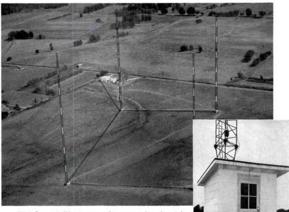
FIG. 6. Four guyed 400-foct towers arranged in a square make up the station's directive antenna array. Phasing equipment for the towers is housed alongside the 10 KW transmitter in a matched panel. The enclosure is standard RCA equipment which is added to transmitters when phasing equipment is employed. Inset shows one of the tower houses located at base of each antenna tower.
