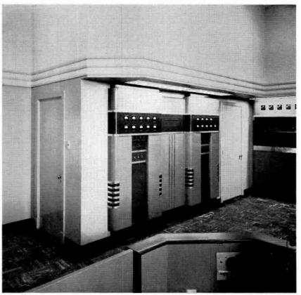
FIG. 4. Above is the 1 KW RCA Type BTA-1L emergency standby transmitter. The unit is mounted flush in a drop wall. Doors on either side permit easy access to the rear of the transmitter for servicing.
