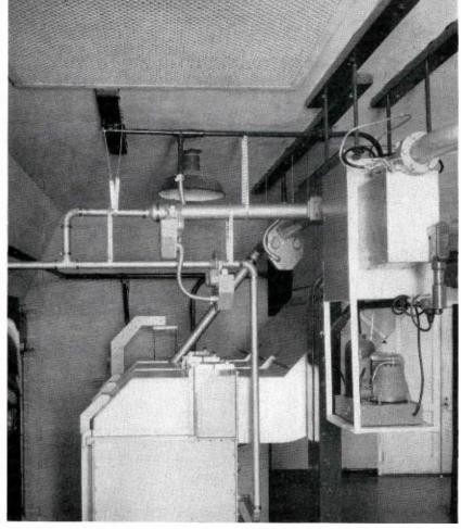
FIG. 8 (above). Closeup of a portion of the 50 KW FM amplifier unit showing the transmissionline power cutback switch arrangement. (Visible in center of photo.) The transmission line monitor and harmonic filter are shown at extreme right.
