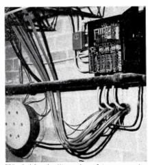
FIG. 7 (above). View of conduit entrance to building, junction box with tower light flasher, photo-electric motor starter, and (at left) reel of surplus scampling line from #2 and #3 towers.
