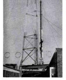
FIG. 2. Four-section Pylon completely assembled is shown here ready to be hoisted up the tower.
