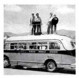
FIG. 5. The KRDO mobile unit is adequately equipped to broadcast almost any event. As shown, the root serves as vantage point for the announcer. The small "dish" is a parabolic microphone.
