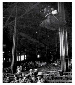
WEW's camera setup is unusual. No. 1 Camera (shown above) is located in a "crows nest" directly behind homeplate and about 20 feet high, which gives an ideal cover shot. No. 2 is in the second tler toward 1st base. No. 3 is mounted like No. 1 in the lower stands opposite 1st base. Latter is used with 25" lens for dugout interviews —thereby saving the work of moving a camera down to the field for this purpose. WEWS telecasts have been much acclaimed by reviewers.
