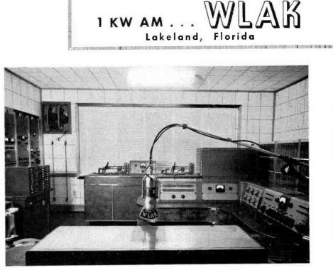
FIG. 3 (above). View from WLAK studio, looking into control room. Visible at rear is the WLAK dual-recorder which employs type 73-B professional unit.
