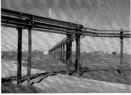
FIG. 6. This is another view of the transmission line branching point. Because separate feed The large line at the top is the concentric line feeding the FM antenna at the top of No. 3 tower.
