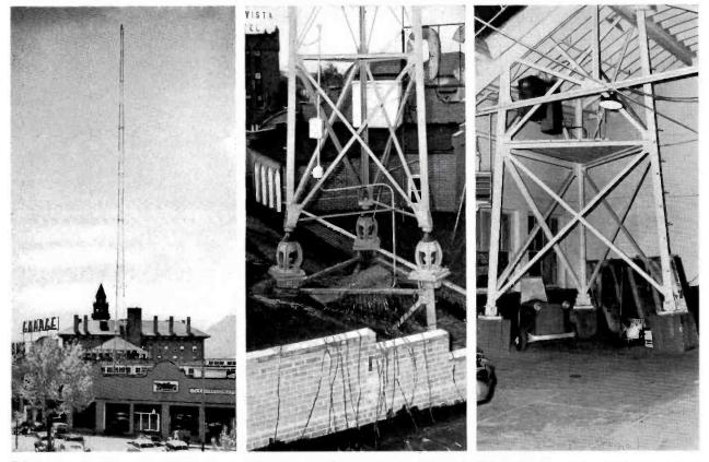
FIG. 1. Tower insulators of the KRDO antenna are located 25 feet above the ground level of a one-story garage.
