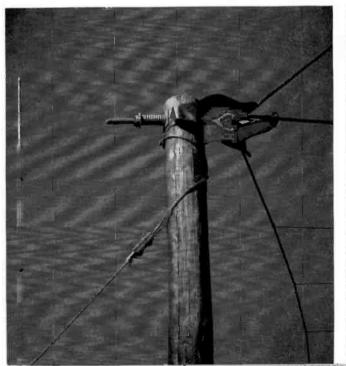
FIG, 10 (below). This is a close-up view of the central ring to which the 120 radials of the elevated ground screen are carefully braised. The ring, in turn, is connected by copper straps to the bonding about the tower base.
