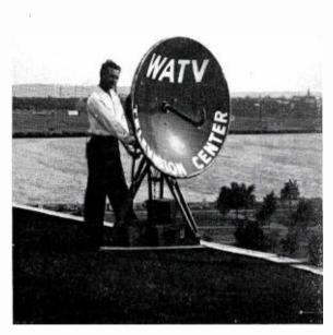
WATV, like nearly all stations telecasting baseball, uses RCA Microwave equipment to relay video signal to studio or transmitter. In many cases roof of grandstand provides necessary height for transmitting parabola.
