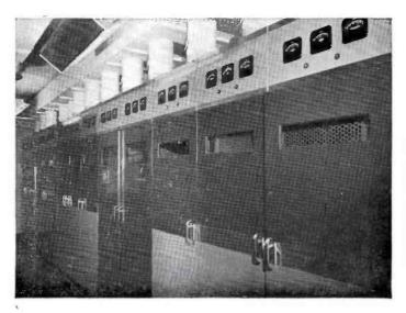
**WENR-TV.** The RCA 5-kw television transmitter Type TT-5A and RCA 10-kw FM transmitter Type BTF-10B at WENR-TV. This ABC station also includes an RCA Superturnstile antenna, field truck and field camera equipment, studio cameras, video and audio controlroom equipment, film projectors, film cameras, turntables, and microphones.
