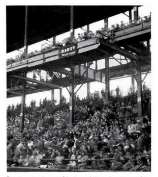
This shows how the special booth was built out from the second tier to provide KSD-TV with its vantage point. All cables and audio facilities are installed permanently to facilitate setup.
