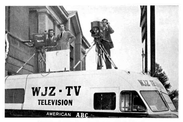
**WJZ-TV.** RCA field equipment in action atop a WJZ-TV field truck. WJZ-TV also uses RCA television camera controls, microwave relay equipment, sync generators, studio cameras, video and audio control-room console, complete film facilities, turntables, microphones, Superturnstile antenna, and the 5-kw transmitter Type TT-5Å.
