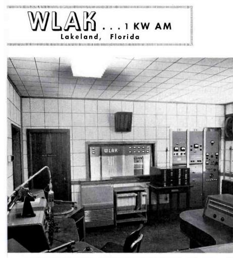
FIG. 1 (above). The WLAK, 1 KW transmitter is visible from window of central control room, Note that monitoring test and audio racks, as well as studio control consoles are all easily reached.
