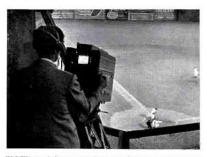
KGO-TV's No. 1 Camera, in a booth high behind homeplate, covers pitched ball—mound to plate—and follows the ball on a hit to show direction before switch to No. 2 or No. 3 to show catch.
