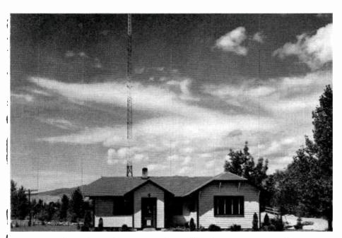
FIG. 1. Shown above is the transmitter building of KXLL which is situated about 200 feet from a river. The antenna tower shown at rear of the building is located at river's edge with half its ground system buried under water.
