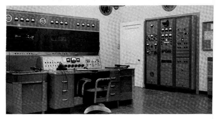
On Thursday, April 14, 1949 KTBS in Shreveport began operation with a new frequency and ten times more power. The new transmitting station operates on 710 kilocycles with a daytime power of 10,000 watts and 5000 watts at night. With these improved facilities, one of the pioneer broadcasting stations of the South will be able to serve better the progressive tristate area of which Shreveport is the center.
