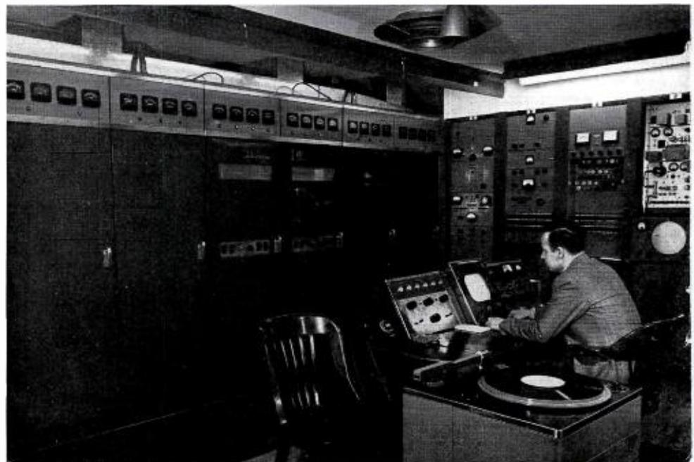
FIG. 3. View inside the transmitter room showing the RCA UHF transmitter, control console and monitoring racks. Transmitting equipment requires little floor space and rivals commercial TV installations in appearance. Seated at the console is Victor Bary, Senior Station Engineer, NBC.
