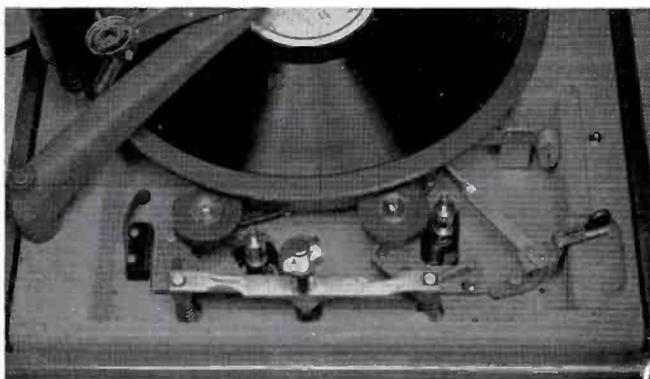
**OFF**—With speed change knob "UP", rubber idlers are moved vertically to low-speed position of drive wheel (note drive wheel has "lo- and hi-speed" shoulders of different diameters). Changing the drive pulleys permits speeds of either 45 and  $33\frac{1}{2}$  or 78 and 45 RPM.
