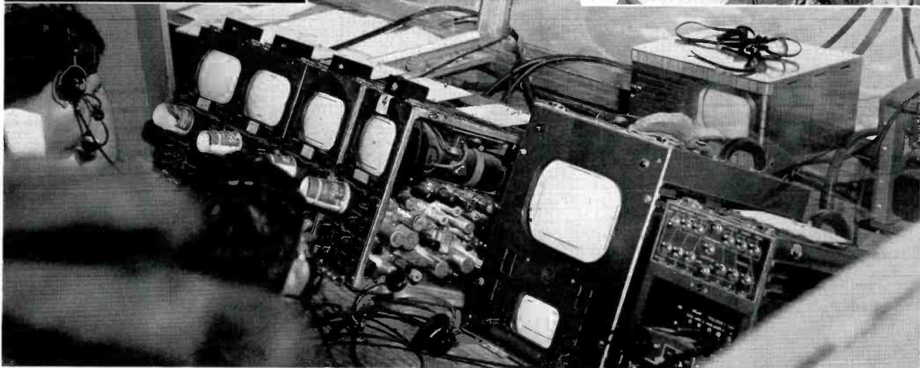
FIG. 14 (above). Closeup of the control room equipment which includes camera monitors, line monitor, field switcher and "Off-air" receiver.
