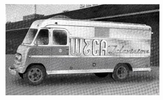
FIG. 58. Overall view of TJ-53A Mobile Unit used to provide complete facilities for remote pickups.
