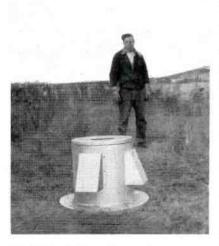
Fig. 9. View of Flange Pedestal Adapter used to mount the UHF Pylon antenna atop the FM Pylon. Wedge-shaped extensions are vent louvers.
