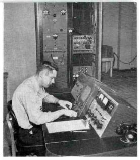
FIG. 8. WSBT-TV Engineer, Howard Paulsen, is shown seated at the RCA TTC-1B transmitter control console. Sufficient blank space is left in the rack to receive a demodulator and sideband response analyzer.
