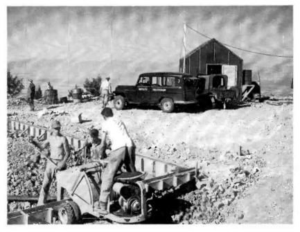
FIG. 4 (right). Another view of the mountain top taken during pouring of the foundations. All the construction materials and equipment were, of necessity, hauled over a temporary road having grades as high as 25% in places.
