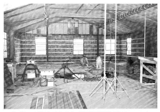
FIG. 5. Interior of the building during construction. All surfaces exposed to outside are covered with 3-incl: fibreglas insulation. The living quarters, which are in the end of the building shown here, have wood floors. The rest of the building has a poured concrete floor.
