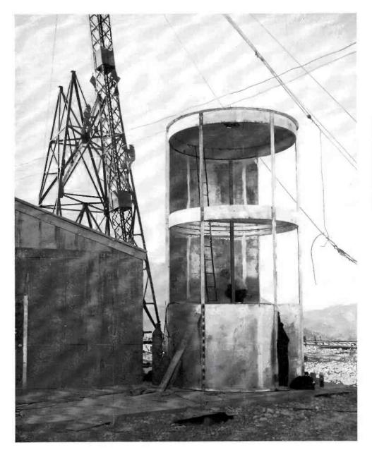
FIG. 9 (leit). A unique feature of the KDYL-TV installation is a microwave "tower", shown here during construction. Two station-owned RCA microwave links provide video circuits from the studios in Salt Lake City. The receiving parabolas are mounted at two levels, as shown in the diagram on the opposite page. The enclosure protects them from the weather and makes maintenance easy.
