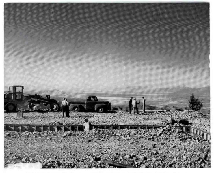
FIG. 3. Before construction could start it was necessary to bull-doze a flat place on the ridge. This is a view looking north from the building site. Southern Idaho is visible in the distance. KDYL-TV covers 87% of Utah, as well as parts of Idaho, Wyoming and Nevada.
