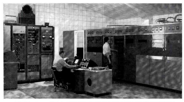
FIG. 8. The transmitter room on Mt. Vision. The RCA TT-5A Transmitter (right) works perfectly despite the rarefied atmosphere. Racks at the left contain video amplifiers, microwave relay receivers and monitoring units. With exception of a few minor units all equipment at KDYL-TV was supplied by RCA.
