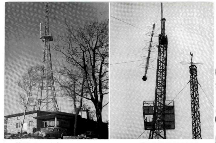
FIG. 3. Two-section heavy duty Pylon passing microwave platform. Constant cross-section of tower from this point to the top is for channel § Supergain Antenna.
