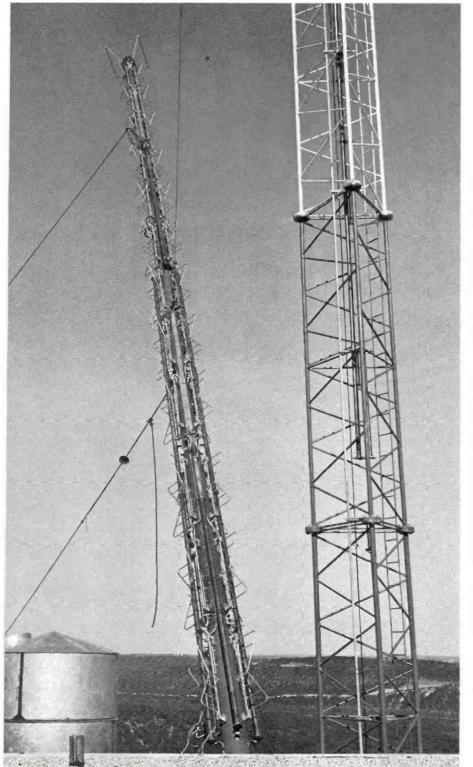
The swift expansion of the television field has brought with it the demand for transmitting antennas in large quantity and at reasonable price. They must be capable of being mounted on towers up to fifteen hundred feet in height and provide reliability under drastic extremes of weather. With an absolute minimum of servicing, such antennas must meet and maintain electrical specifications as rigid as those placed on many types of laboratory equipment operating under controlled conditions.
