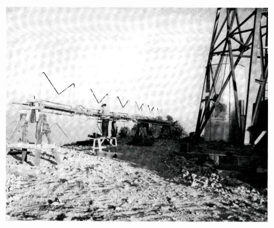
FIG. 2. Assembling the RCA six-bay turnstile at the KDYL-TV site. The base of the specially-built extra-heavy 100-foot tower on which the antenna is mounted is at the right. The microwarve receiving antennas are enclosed in the silo-like structure behind the tower. Everything used at this very exposed site had to be of very heavy construction. The fact that the standard RCA turnstile antenna stands up under such extreme contions is an indication of its high reliability.
