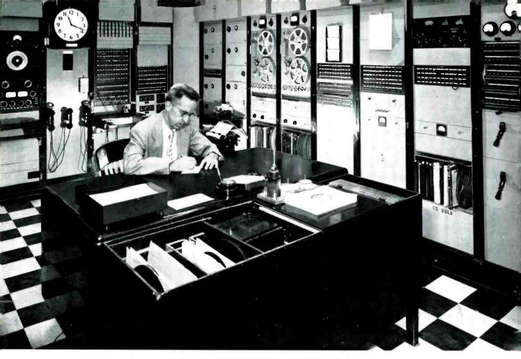
E. B. Landon, Assistant Studio Supervisor of Radio Station KDKA. Pittshurgh, Pa., seated at desk in master control room. The two rack-mounted tape recorders are RCA Professional Type RT-11.
