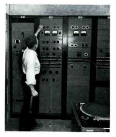
telephone lines and studio equipment is mounted in the wall. Control room windows are five feet above the studio level to provide a better overall view.
