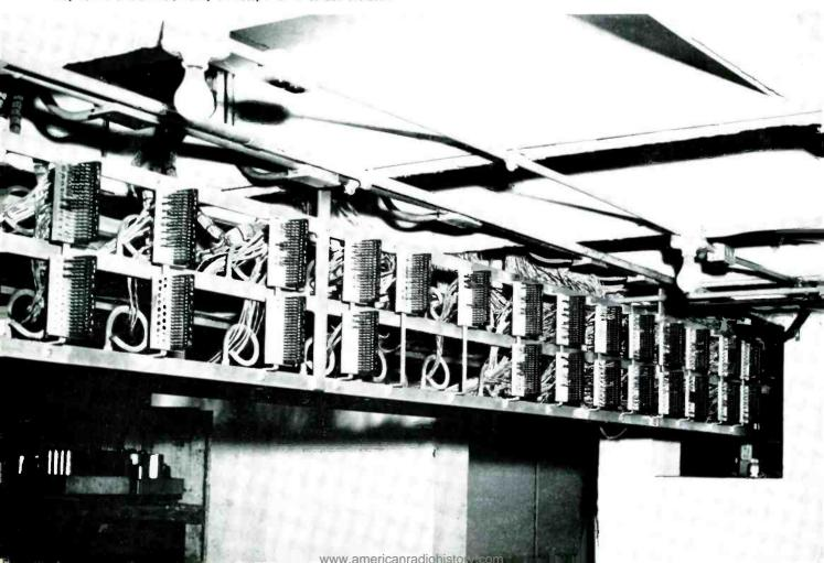
FIG. 2 (right). All of the WBAP racks were wired in the RCA plant at Camden. Cables to terminal boards were made about three feet longer than usual. After racks were set in place at WBAP the terminal boards were dropped through holes in the floor and mounted on a frame in the basement as shown in Fig. 1.
