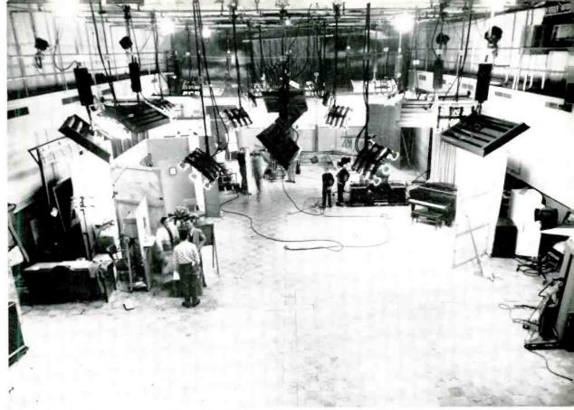
FIG. 9. This view shows the opposite end of WBAP Studio  $\pm 1$ . All lights are suspended from a pipe framework and can be rotated by means of rope controls which are operated from a "lighting bridge" (extreme right in this picture). In normal operation a number of "sets" are crranged along the sides of the studio. Cameras, operating in the center area, move from set to set.
