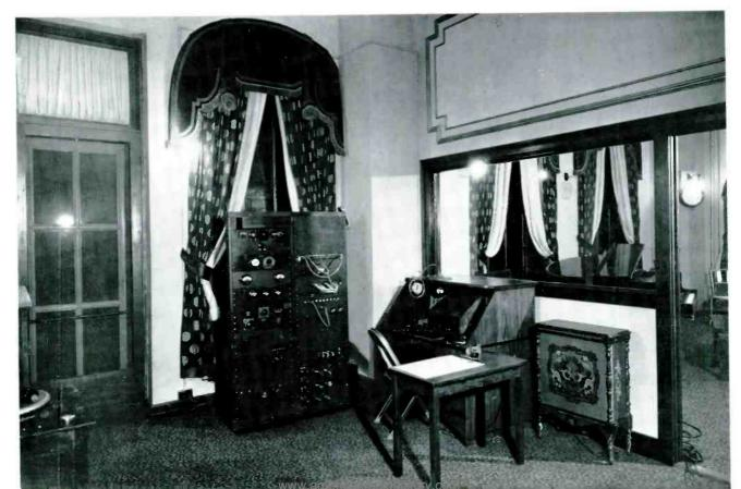
FIG. 14 (right). This was the WHBQ 250-watt control room in the Hotel Gayoso, with its 76-B console, 70-C turntables, 64-B loudspeaker and 40-C amplifier mounted in the rack at right. To the right is the original small studio, later converted to a control room. To the left is the large studio. WHBQ outgrew these facilities, moved to the Hotel Chisca January 9, 1953.
