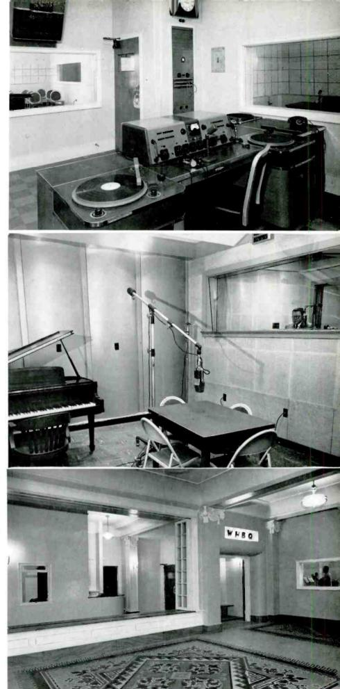
FIG. 15 (center). This view of the latest large studio shows the junction of the polycylindrical diffusers with a blanket wall under Transite. A part of the serrated ceiling is also visible. The control room at the right has a full view of the entire studio.
