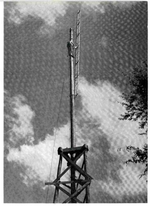
FIG. 4 (right). The transmitting antenna for the bccstor station is a vertical zig-zag type with a power gain of 19.4 db. It is mounted on a 90-loot pole about 100 feet from receiving antenna site.
