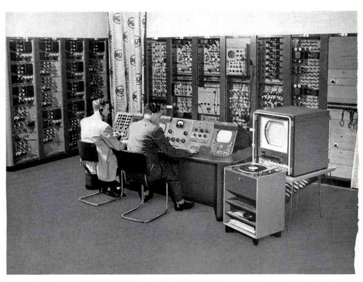
FIG. 5. Control center for the entire exhibit. All operative equipment was controlled from this point—3-Vidicon Color Film Chain, Monochrome Vidicon Film Chain, Color Studio Camera and complete audio and video switching for various viewing locations throughout the exhibit area and other points in hotel.
