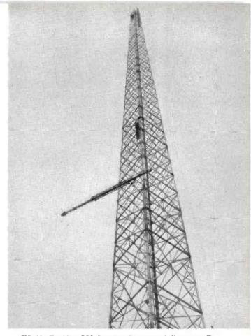
FIG. 13. The 6-bay RCA Superturnstile antenna half way up. The antenna was placed on top of a 441-foot Lebigh tower making the overall height of 480 feet.
