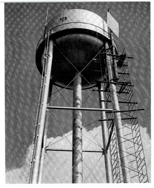
FIG. 2 (right). The receiving antenna for the booster station is a zlg-zag type with a gain of 20.5 db. It is mounted on a 100-foot water tower at a site about two miles northeast of the center of the city. (See Fig. 3.)
