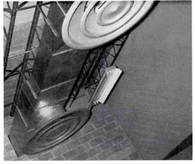
FIG. 3. Ventilating and air conditioning system installed in ceiling of main studio. A large volume low velocity air system is used in order to reduce noise from air turbulance. The inside areas of all ducts are lined with a 1-inch blanket of spun glass insulation which has aided in reducing blower noise.
