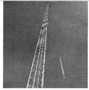
On its way up, the WFAA-TV Channel 8 antenna is carefully quided towards the corner of the triangular tower which it will occupy.
