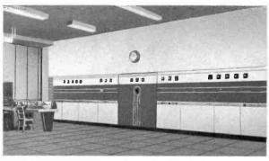
RCA 50-KW Shortwave Transmitter using RCA-857B high-power mercury-vapor rectifiers
