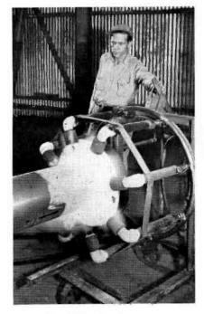
Jig welding of a flange on a round tower leg member by means of a jet welding device.
