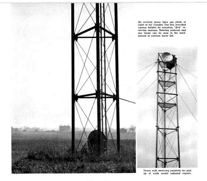
site was already in existence at RCA. The site consisted of cleared terrain with a rotating pedestal for the scale model antennas, and a tower located at a distance of 1400 feet from the receiving equipment. A shallow valley between the pedestal and receiving tower aided in minimizing ground reflection effects.
