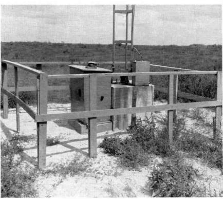
Base of tower with line terminating unit (left) and tower lighting choke (right).
