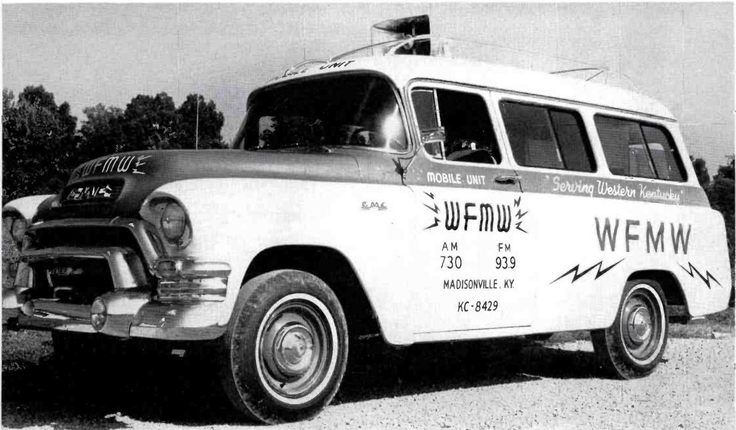
FIG. 1. Mobile unit remotes are relayed to station via 450-mc broadcast relay band.
