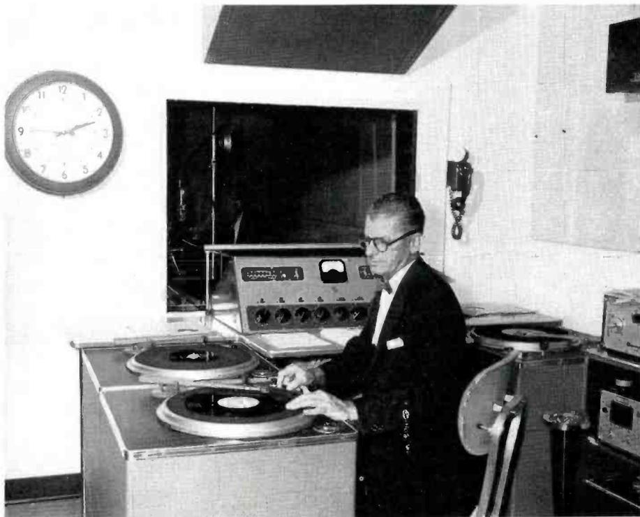
FIG. 7. Studio "B" control room is typical of the facilities available in the other two control rooms and contains a BC-2B Studio Console, three BQ-2A turntables, tape recording equipment and LC-1A monitor loudspeakers.
