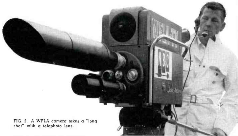
FIG. 2. A WFLA camera takes a "long shot" with a telephoto lens.
