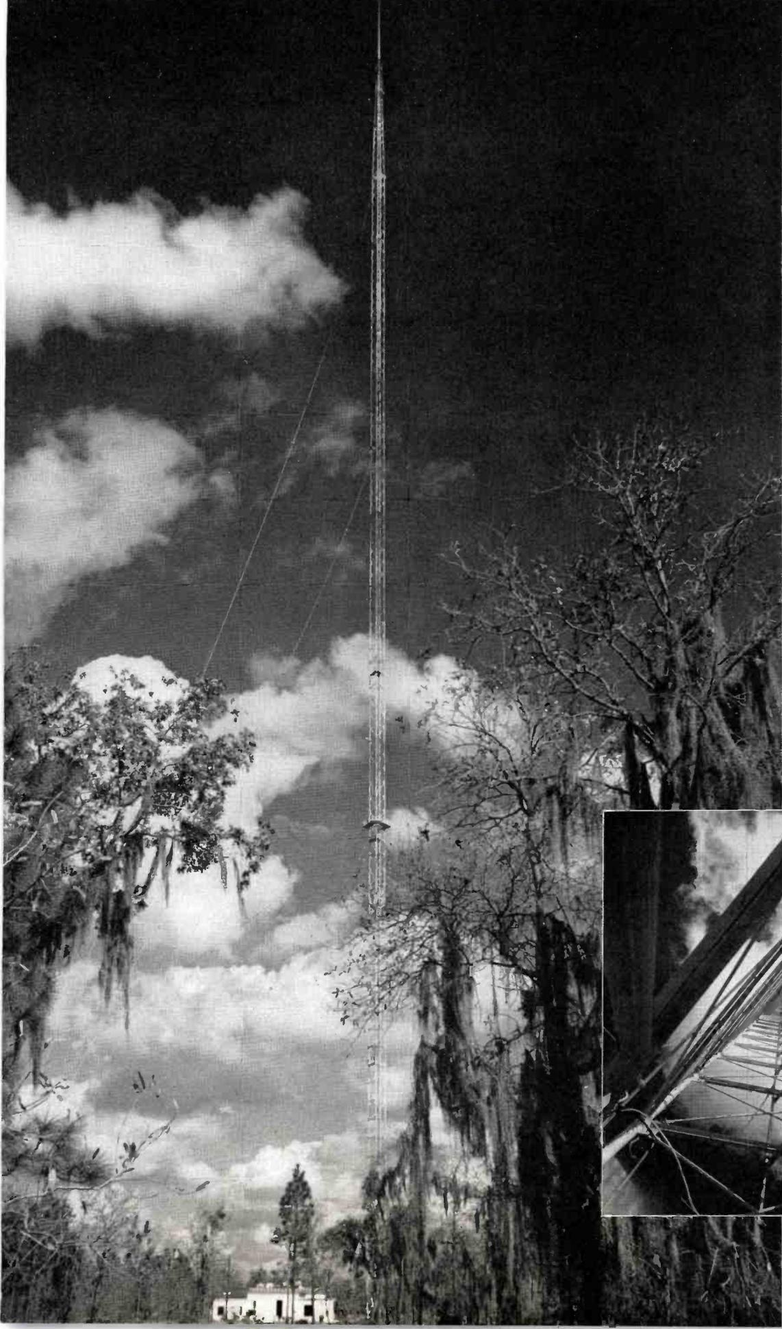
FIG. 25. WFLA-TV tower and antenna point 1055 ft into Florida skies. The Ideco tower structure supports an RCA TF-12AH twelve-section superturnstile antenna. Looking through a picturesque setting of trees bearing Spanish Moss, the transmitter building is visible at the base of the tower.
