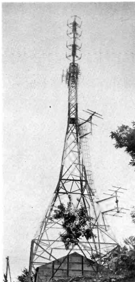
FIG. 22. Typical RAI automatic repeater (translator) for FM and TV at Brunate in Northern Italy.
