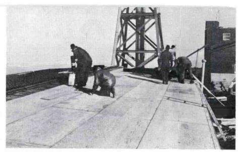
FIG. 16. Prefabricated plywood panels are set in place in the first stage of reinforcing the transmitter house roof.
