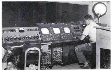
FIG. 30. Equipment arrangement in the control room allows RCA TC-4A switcher to be used for one main operation during periods of network and film only. FIG. 31. Two separate TK-21 monochrome film systems, each equipped with a RCA TP-6 projector, provide utmost reliability in daily operation.
