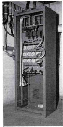
FIG. 8. Camera patch panel in Army Hospital is used to connect TV cameras in operating suite with control room.
