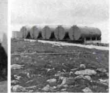
FIG. 10. WMTW's tuel is stored in five 20.000 gallon tanks. These tanks hold a full year's supply of fuel.
