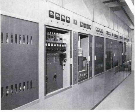
FIG. 7. RCA TT-25AH Transmitter as installed in the transmitter room. Ductwork cannot be lixed to the ceiling because of extreme wind velocity, often moves the building as much as 4 or 5 inches.
