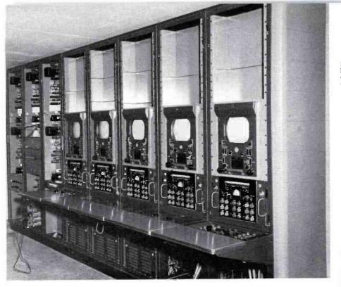
FIG. 16. Three-channel distribution system uses RCA Monitrans. This enables viewer to choose from three programs at any location.
