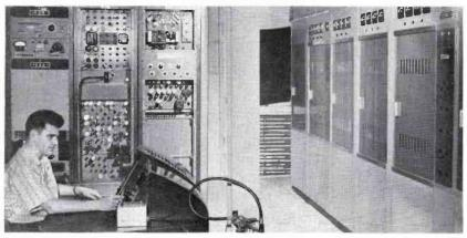
FIG. 8. View of WMTW's 25-kw transmitter showing control and auxiliary equipment. Deflection and amplifier chassis for TK-21 vidicon camera chain are mounted in the center cabinet rack.
