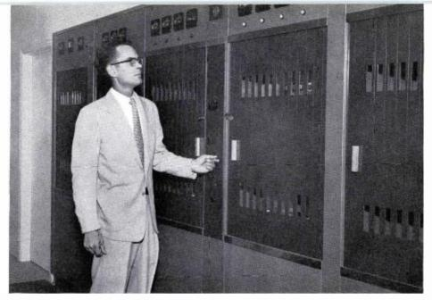
FIG. 7. The author is shown at the BTA-10H 10.KW Transmitter. An adjacent phasing cabinet matches the output of the two towers in the array.
