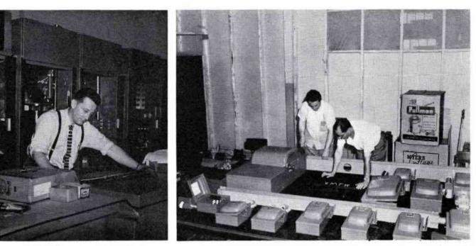
FIG. 11. Chief Engineer Parker H. Vincent supervises preassembly of transmitter equipment.
