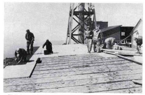
FIG. 17. End grain balsa sandwiched in plywood is added as a shock absorber.
