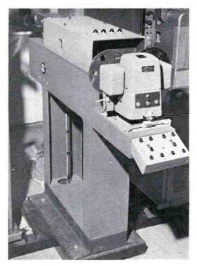
FIG. 11. Composite remote control for film and slide projectors.
