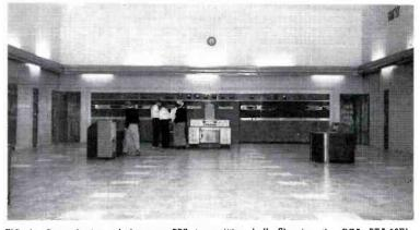
FIG. 4. General view of the new BBS transmitting hall—Showing the RCA BTA-50F1, medium wave transmitter, control console and monitoring loudspeaker. The transmitting hall also houses two RCA BHF high frequency transmitters, with provision for two more.
