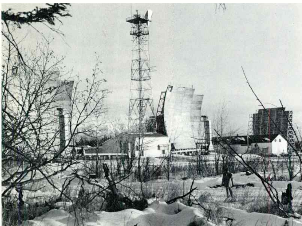
Old and new in Alascom's telecommunications. Microwave towers like the one at left are replacing earlier signal reflectors (to the immediate right of the tower).
