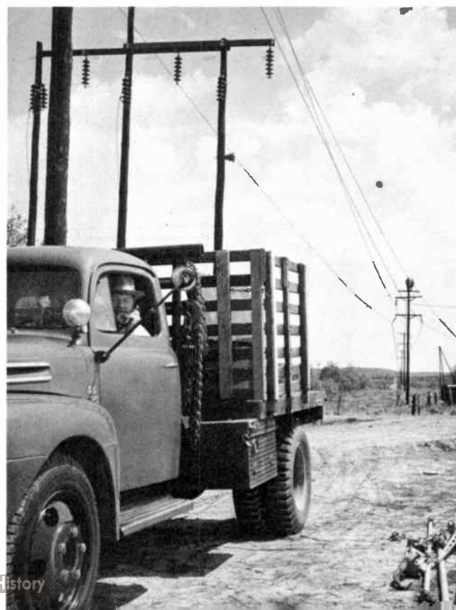
Substation Foreman coordinates work of several crews
