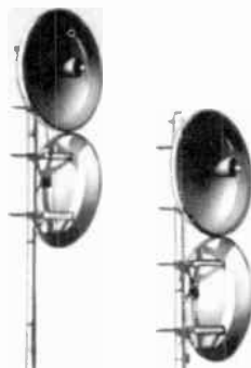
Fig. 3—Antenna arrangement on the roof of Steam Electric Generating Plant showing parabolic reflector placement to facilitate parallel signal paths.
