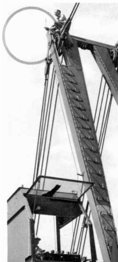
"Carfone" radio antenna is only 18 inches long but gives coverage of more than 300 square miles
