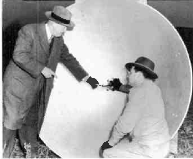
Paul Godley, Consultant for the turnpike (left), Earle Whitaker, RCA Service Company, examine "dish" reflector
