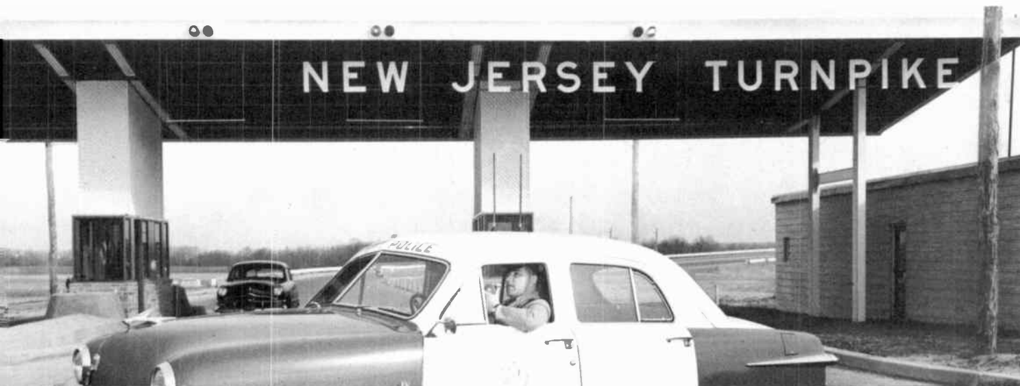
Each tollgate on the turnpike is radio-equipped and ties into communications system
