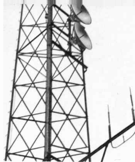
Directional antennas on mobile units and station towers provide effective coverage of turnpike with minimum "spill-over" into adjacent areas
