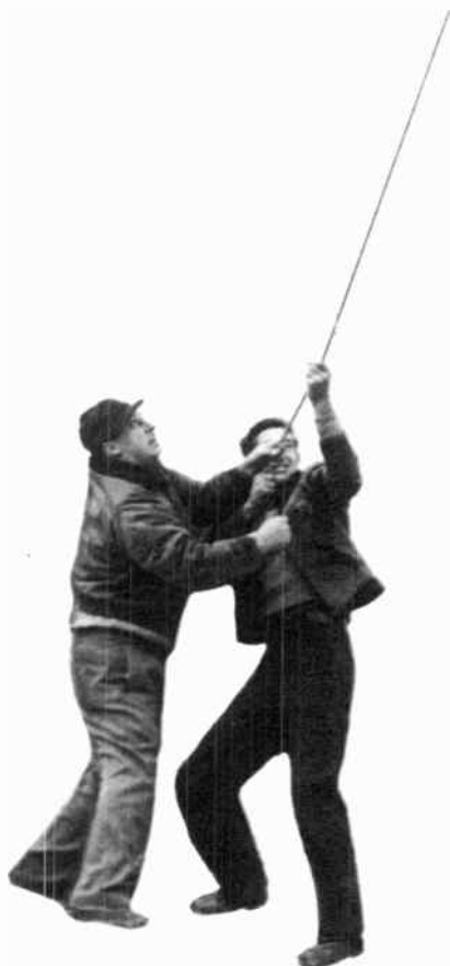
Riggers strain at tackle as huge microwave antenna and reflector go skyward
