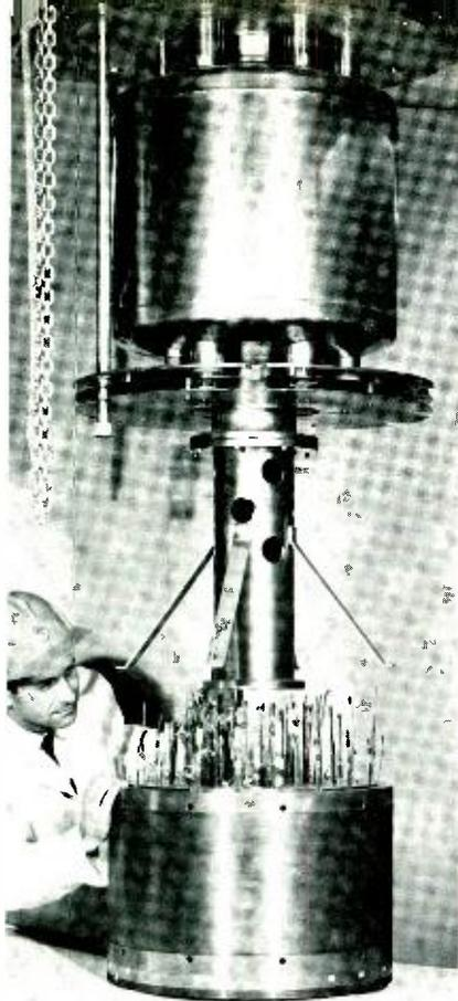
Fig. 13—Six-inch-bore, 140-kilogauss magnet.
