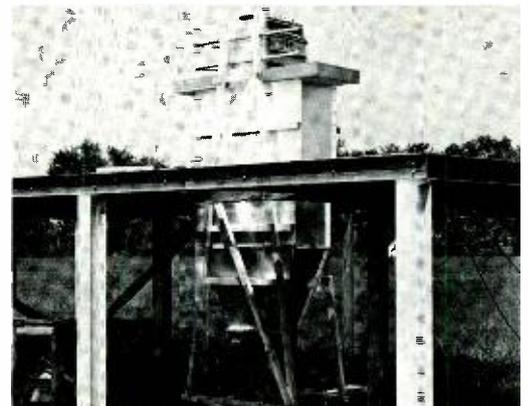
Fig. 11—Photograph of 100-element transfer array in test configuration.
