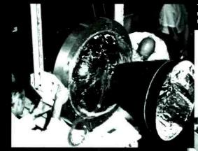
The South panel, containing the 24 transponders, was assembled and tested by RCA, Ltd. Here, AED technician Bob Parsons is shown preparing the transponder subsystem to mate with the spacecraft.
