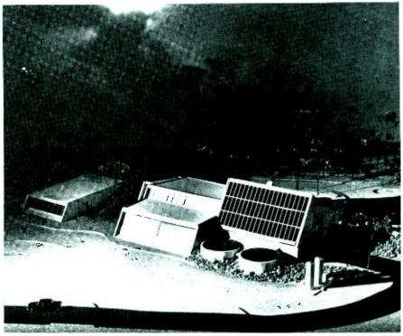
Fig. 1 — A highly energy-efficient wastewater treatment plant planned (by Wright, Pierce, Barnes and Wyman of Topsham, Me.) to use passive solar heating through large, all-south-facing windows, active solar collectors (dark panels), methane storage, heat pumps, etc.
