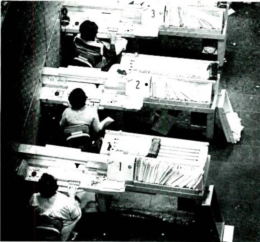
**Postal Sectional Centers and Area Distribution Centers contain letter sorting machines.** In these machines, unsorted letters are mechanically moved to a position in front of an operator who keyboards address data. This keyed data causes the letter to be moved to a correct output sort bin. Re-sort at several locations is typical for a letter traversing the country.
