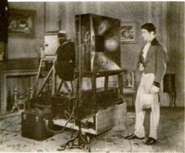
Further advances in television were revealed in 1932 when field tests of 120-line television were made by RCA at Camden, with signals relayed by radio from New York through Arney's Mount, New Jersey. The novel feature of this test, conducted on May 25, was that the pictures were automatically relayed for the first time, thus giving rise to the promise that such relay stations might some day dot the countryside
