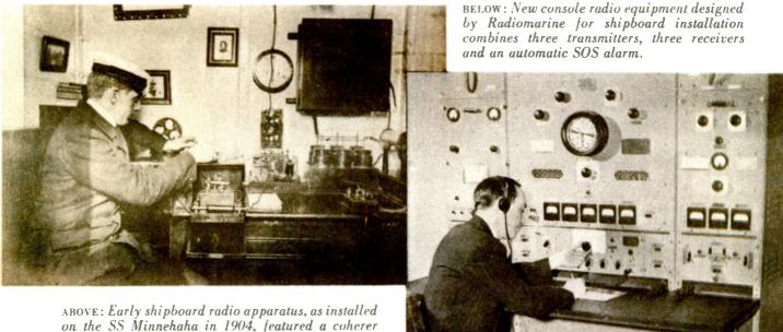
with tape recorder and a spark-coil transmitter — a marked contrast with the modern, compact marine apparatus which utilizes electron tubes and establishes communication with land from any latitudelongitude on the Seven Seas.
