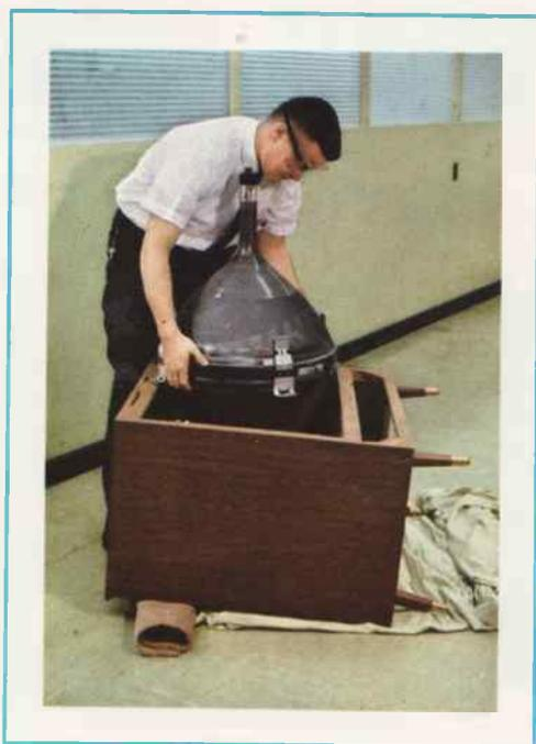
**FIG. 10-4.** Lifting the color picture tube out of the cabinet.
