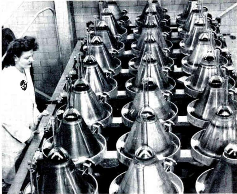
*The faces of the RCA 16-inch television tubes receive a fluorescent coating on which the electron beam "paints" the picture.*
