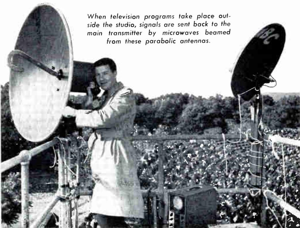
*When television programs take place outside the studio, signals are sent back to the main transmitter by microwaves beamed from these parabolic antennas.*
