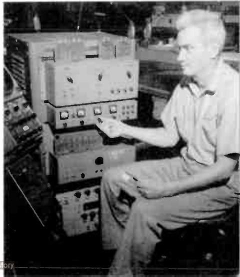
Harold Conaty shown operating the RCA-ARQ Register Checking Unit which he and Anthony Falco designed and built. The unit saves time and material in shop maintenance work and proved to be a valuable contribution to the company operations.
