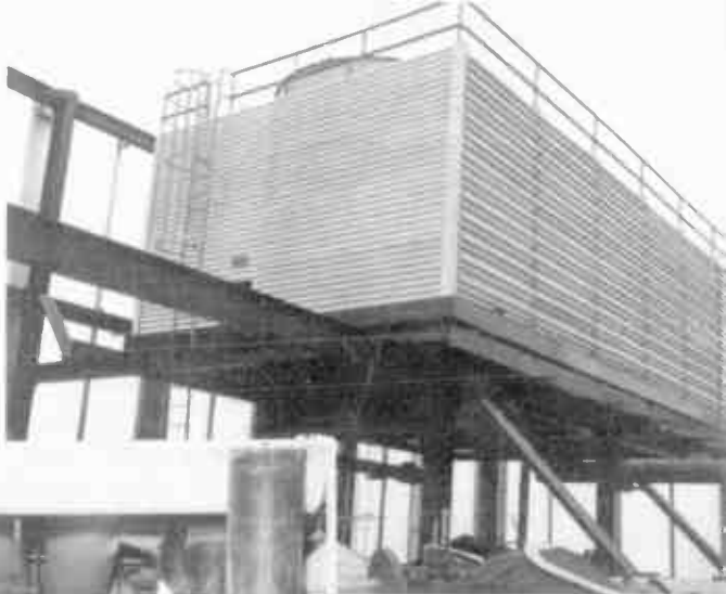
Cooling tower on roof. Three 25 h.p. exhaust fans cool water for re-entry into cooling system.
