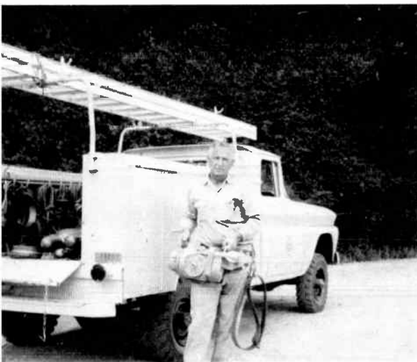
Cable splicer Roy Pepper holding the spinning machine used for securing the cable to the messenger.
