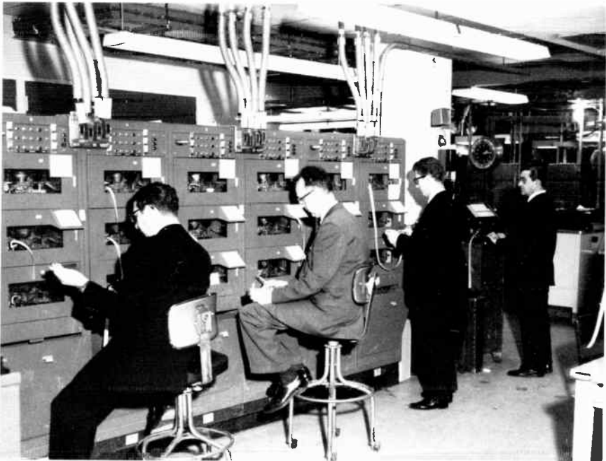
Section 3. These new consoles receive message telegrams from overseas. As the messages are received in tape form the operators scan them, insert the tapes into pneumatic tube slots above the console for dispatch to their destination point on the operating floor.
