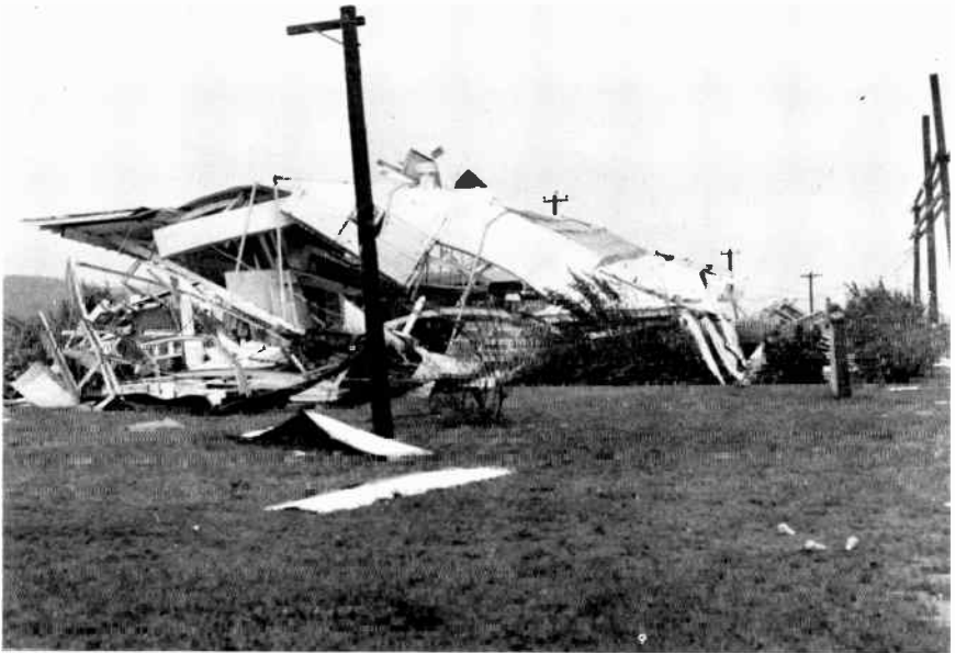
Lashed by 175 mph winds with gusts up to 200 our transmitting building at Barrigada was disintegrated. This photo was taken shortly after Karen passed over the site.
