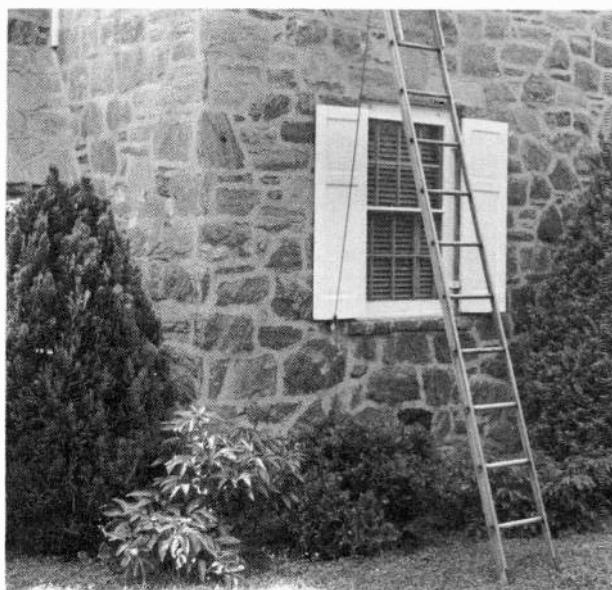
Do not set up the ladder directly in front of a window.
