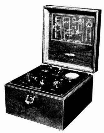
Figure 16-180 K.C. Test Oscillator
