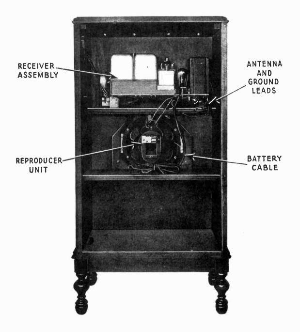
Figure 1-Rear interior cabinet view of Radiolu 22
