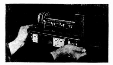
Figure 26-Removing receiver chassis from cabinet
