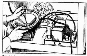
Fig. 13-CenteringCone in Electro Dynamic Reproducer
