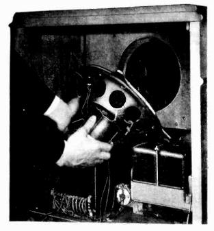
Figure 26—Removing reproducer unit from Radiola 46
