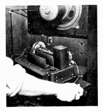
Figure 31—Removing receiver chassis and shelf from cabinet
