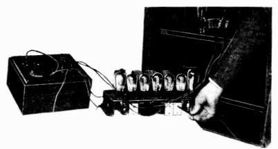
Figure 15-Method of adjusting oscillator trimming condensers
