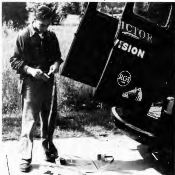
Assembly of the chimney bracket is a ground operation!
