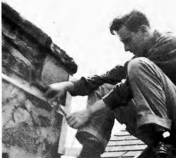
Make sure that the strap is level around the chimney.
