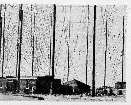
This Marconi radio transmitting station erected at Wellfleet, Mass., in 1902 succeeded in sending signals across the Atlantic.
