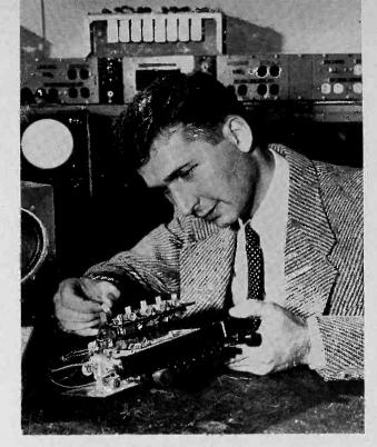
A boon to motorists is this automobile radio, operating from transistors instead of tubes. The transistors operate directly from a 6-volt car storage battery.
