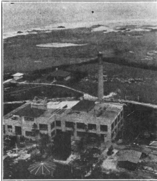
POWER HOUSE—OCEAN, IN BACKGROUND
