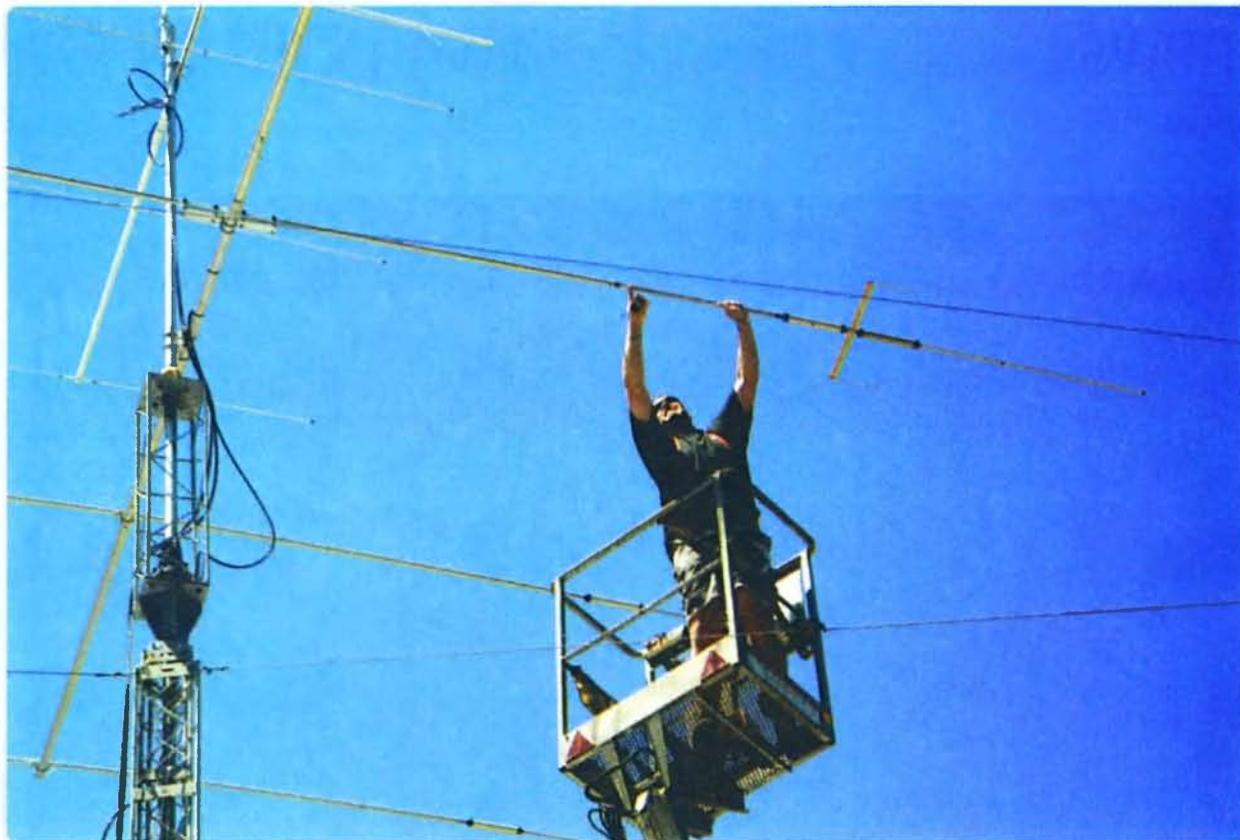
Photo 2: Maintenance work at the HARG. Heath VK6TWO installs the 40 metre traps on the HARG beam.
