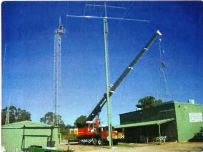
Photo 2: The principal antenna mover, the crane, in the operating position.
