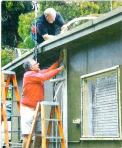
Photo 1: SPARC members working on the split air conditioning system.
