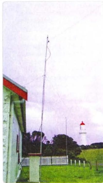
Photo 2: The HF antenna outside the keeper's cottage.
