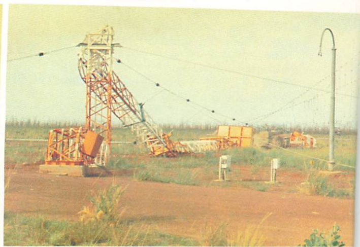
One of the masts on the ground following the cyclone damage.
