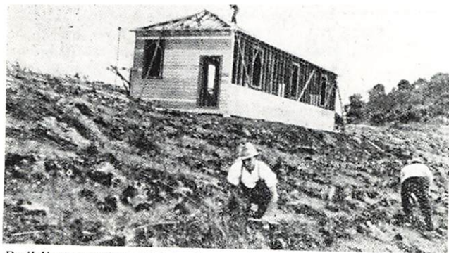
Building erection and earth mat installation Radio Hill 1926
