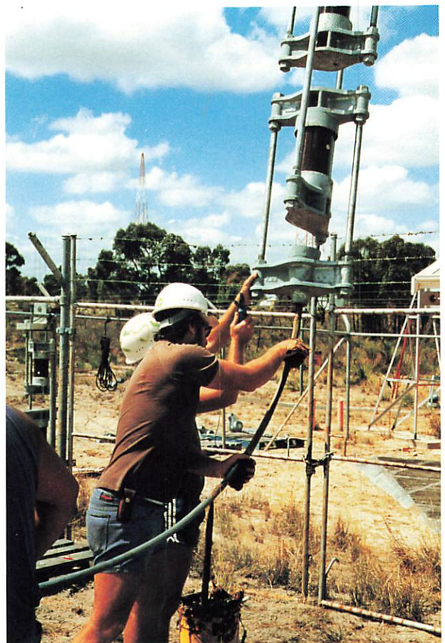
Applying protective grease to guy rope.
