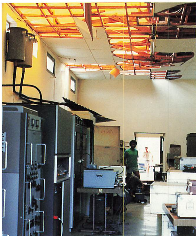
Damage to ceiling and roof of transmitter building.
