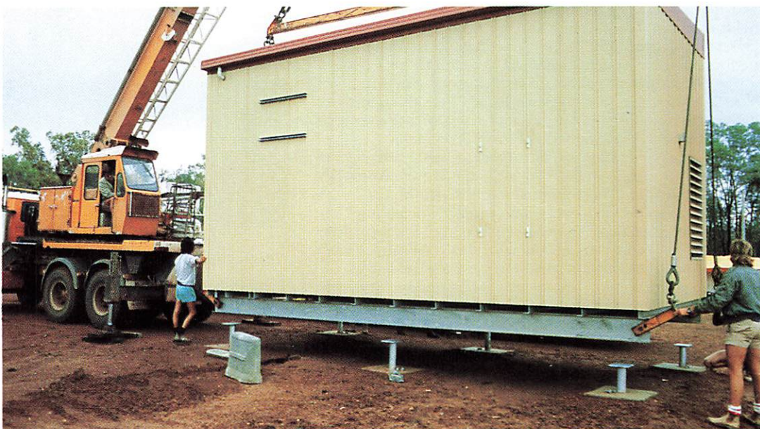
Transmitter building being placed in position - 4CH.
