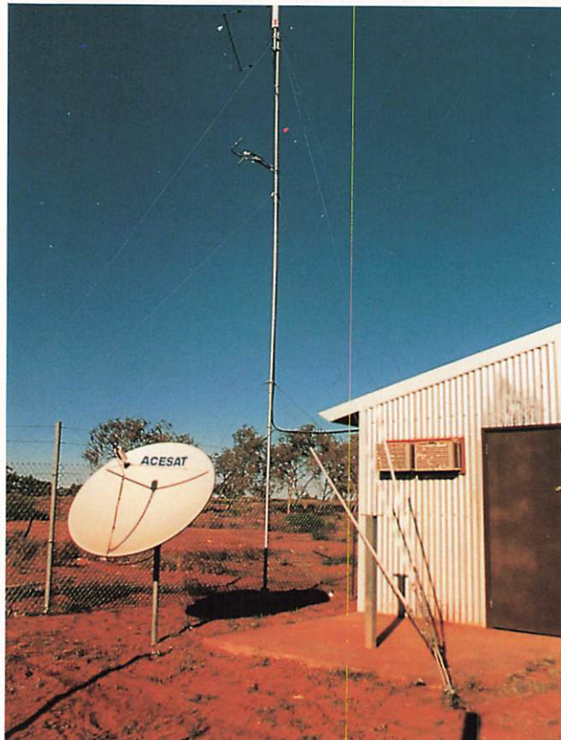
1.5m dish and mast with TV and FM antennas alongside equipment hut
