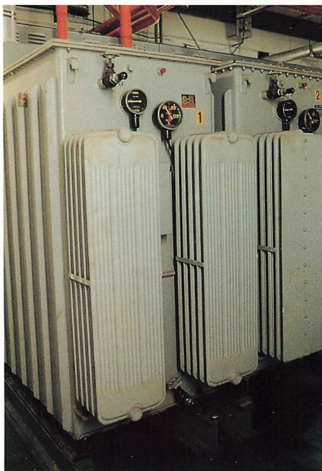
Typical oil filled transformers 250kW transmitter
