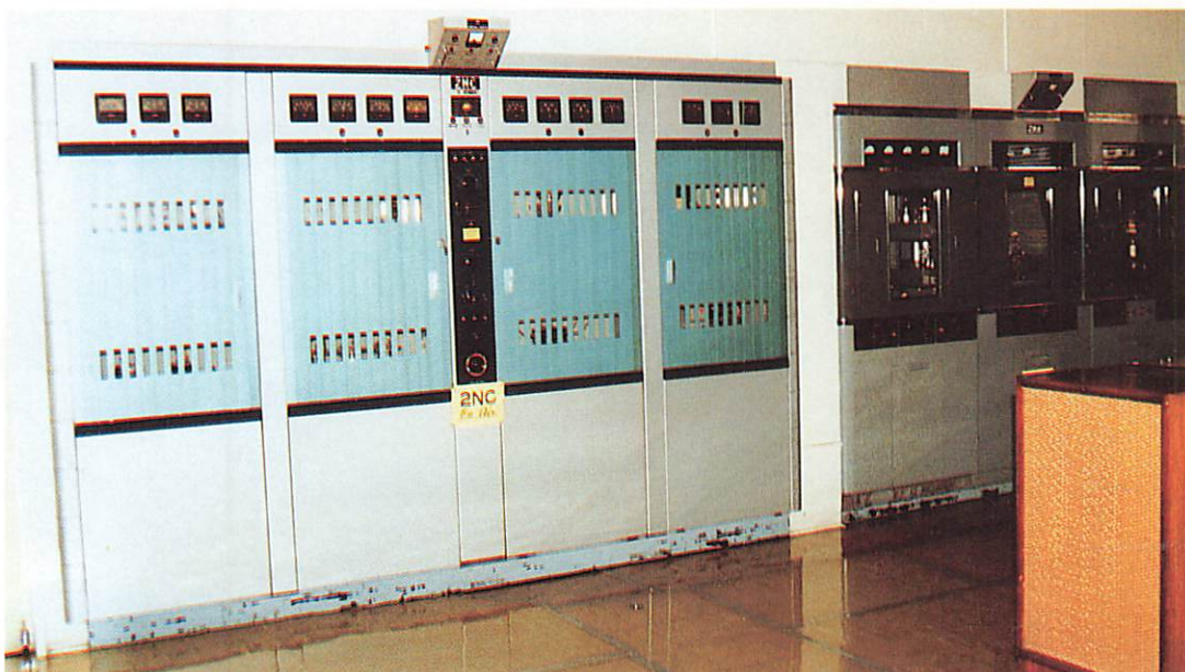
Main transmitter – 10kW on left.
