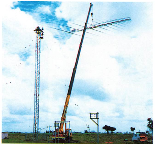
Log periodic antenna being re-erected following repair.
