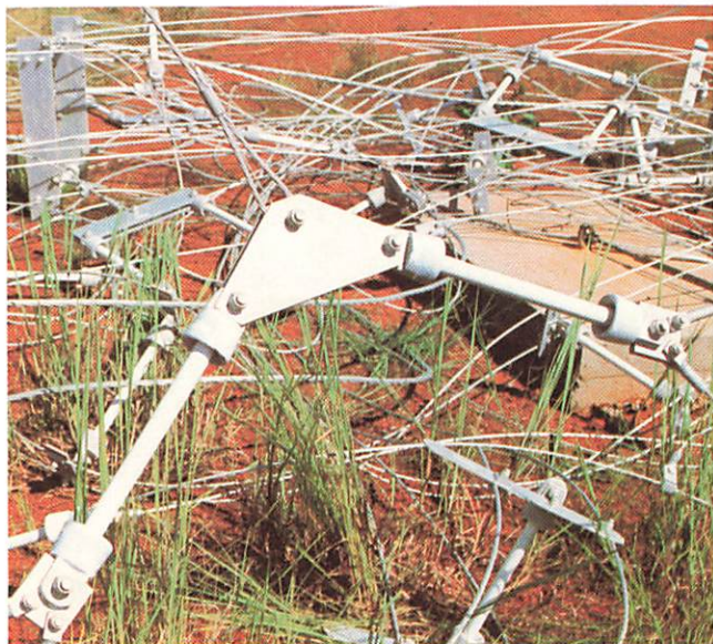
Antenna bunched on ground after being lowered.
