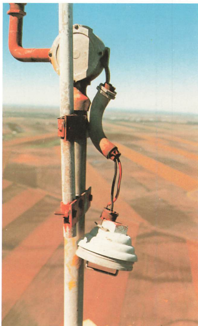
Damaged mast lamp fitting.
